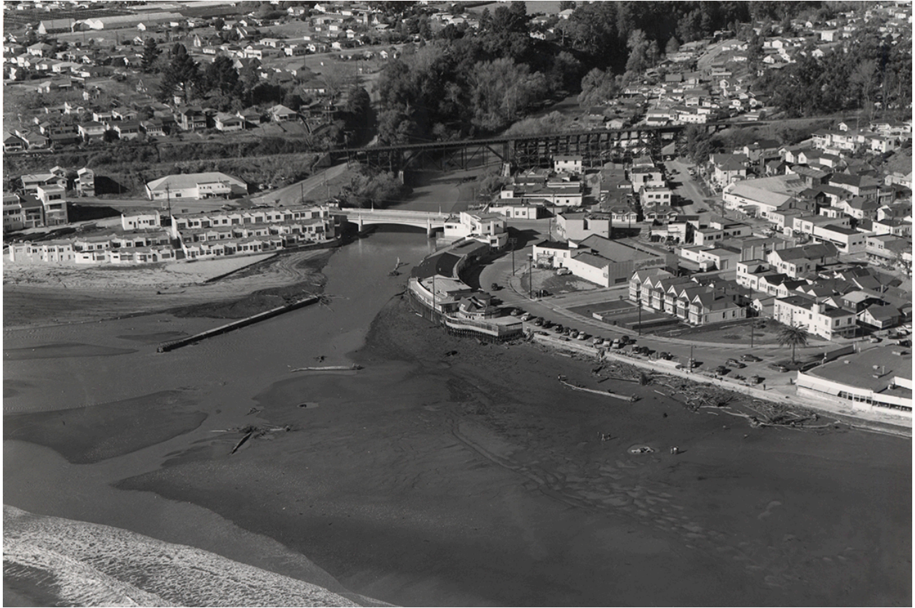
Post-World War II Soquel Creek Estuary at very low tide (present-day Stockton Bridge with flume exposed on the beach after the December 1955 flood). Riparian corridor re-established on west side above Stockton Bridge since 1931 photo; circa 1955-56 after the flood. (Courtesy of the Capitola Historical Museum)
