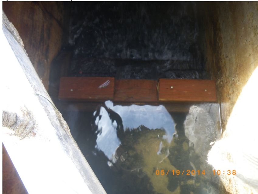
Reconstructed Weir Inside the Flume, 19 May 2014
