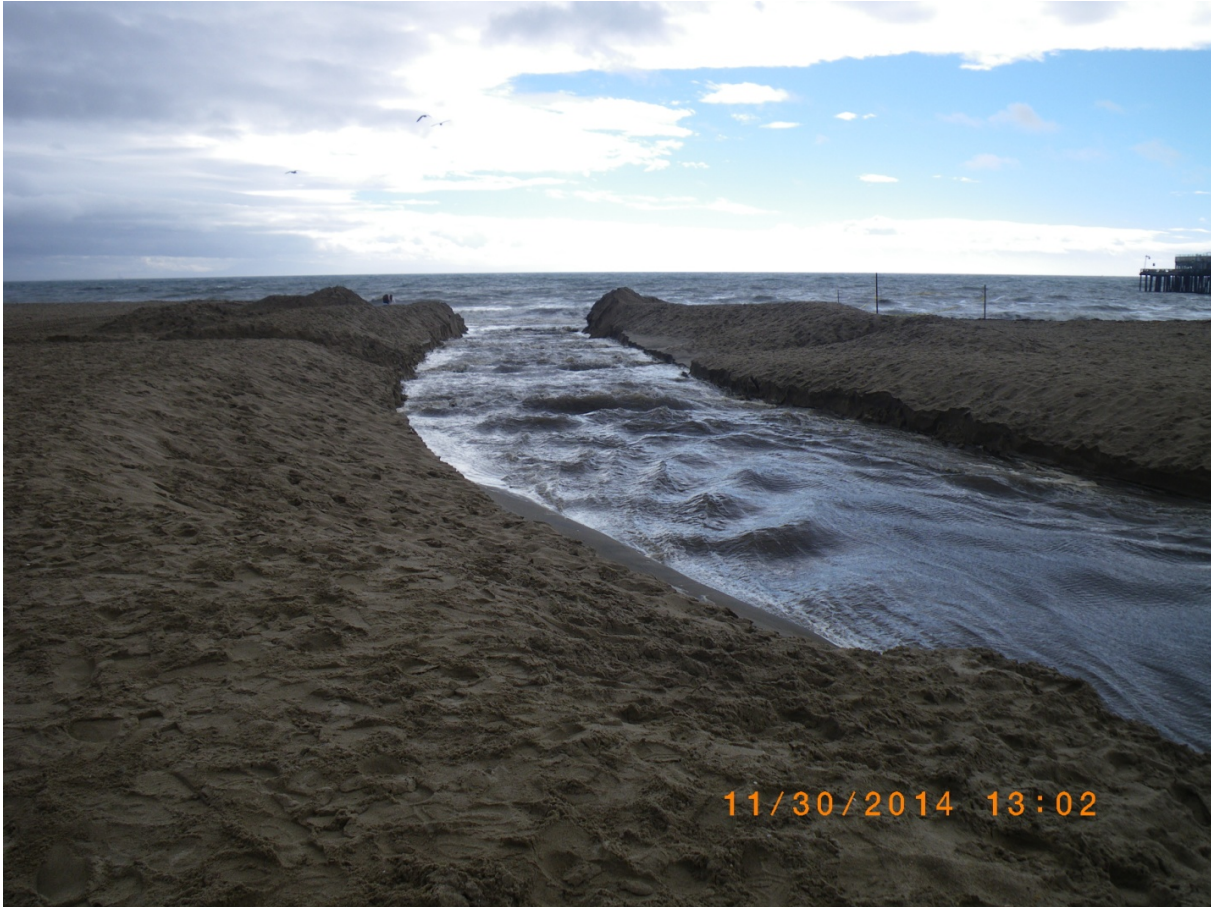
Outlet channel through beach after an emergency breach on 30 November 2014. (Time printed on the photo was 1 hour later than the actual time of 1202 hr.)
