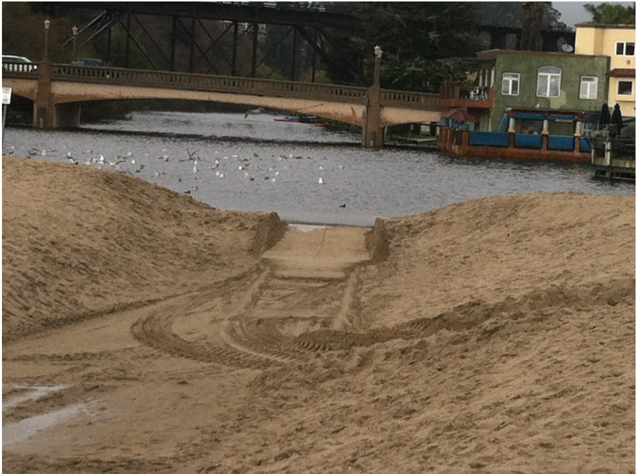
Inner Berm being overtopped at 1115 hr on 30 November 2014
