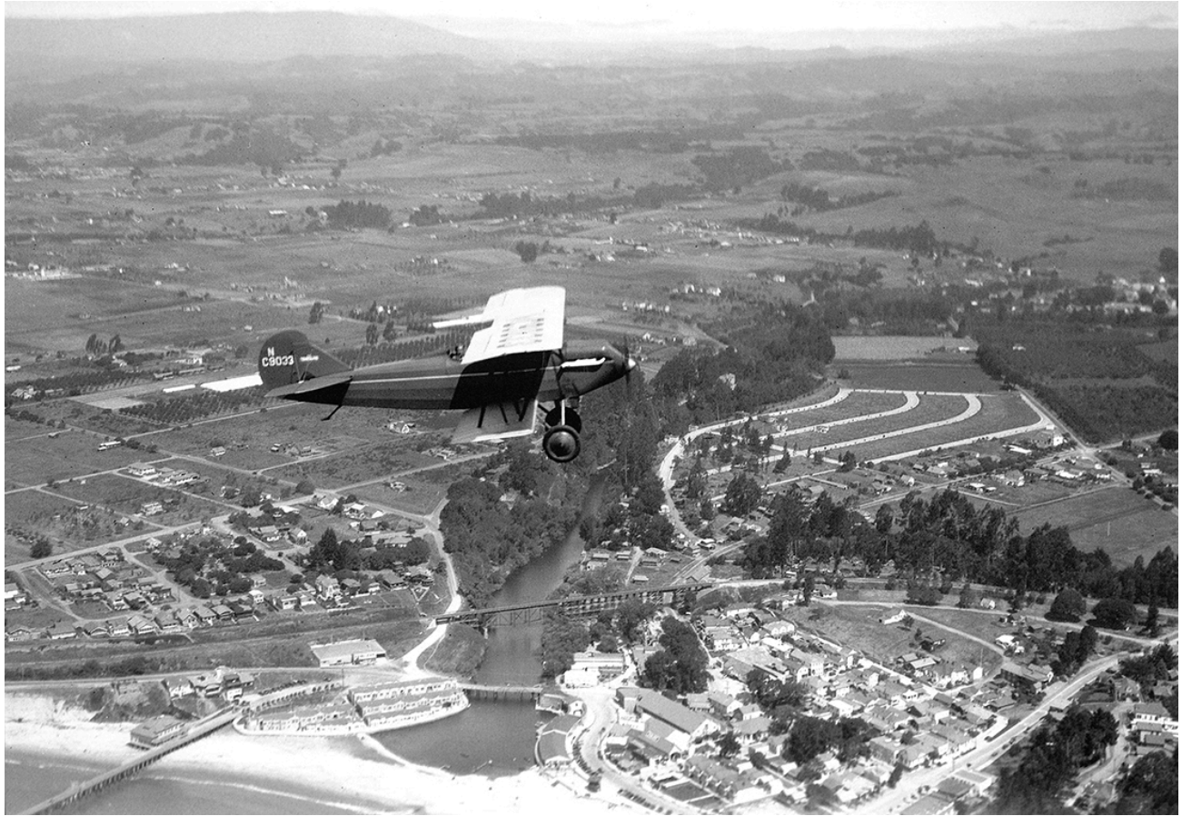
Soquel Lagoon Post-Venetian Court Construction- Older Stockton Avenue Bridge and prior to expanded development on eastern margin of the Lagoon, above and below the Railroad Trestle; circa 1931.
