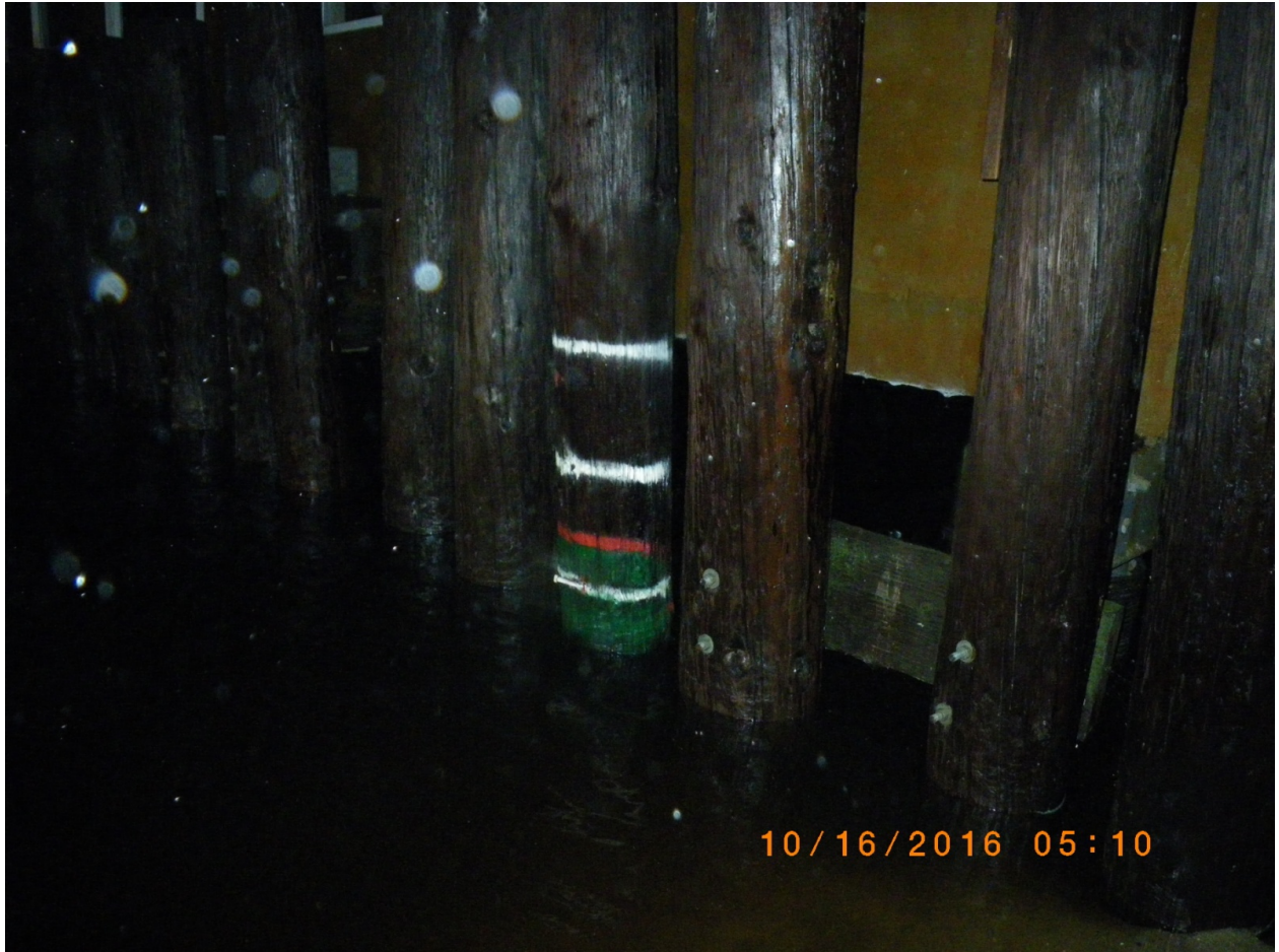
Lagoon water surface shortly after the facilitated breach (red line indicated point of flooding). 16 October 2016
