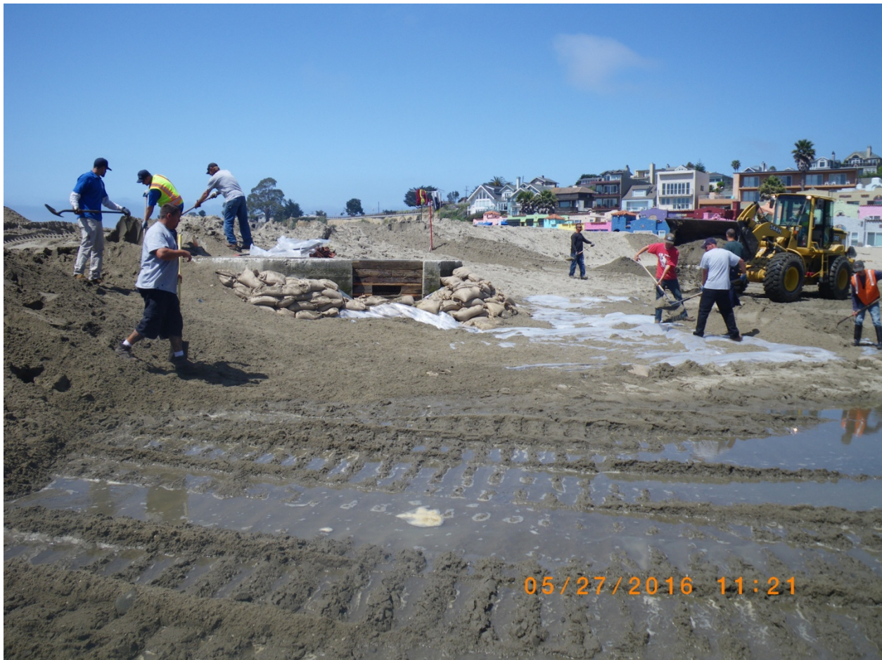
Preparation of the flume inlet.
