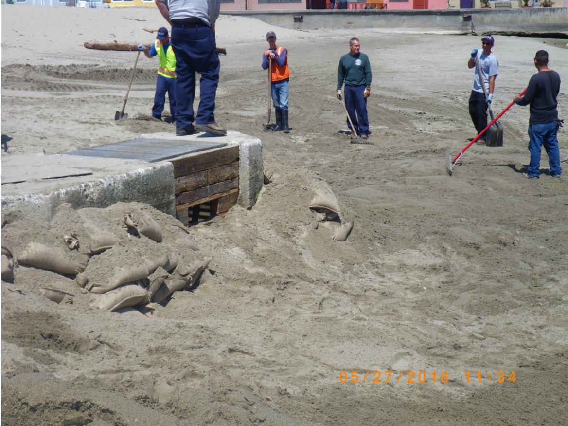
Preparation of the flume inlet.
