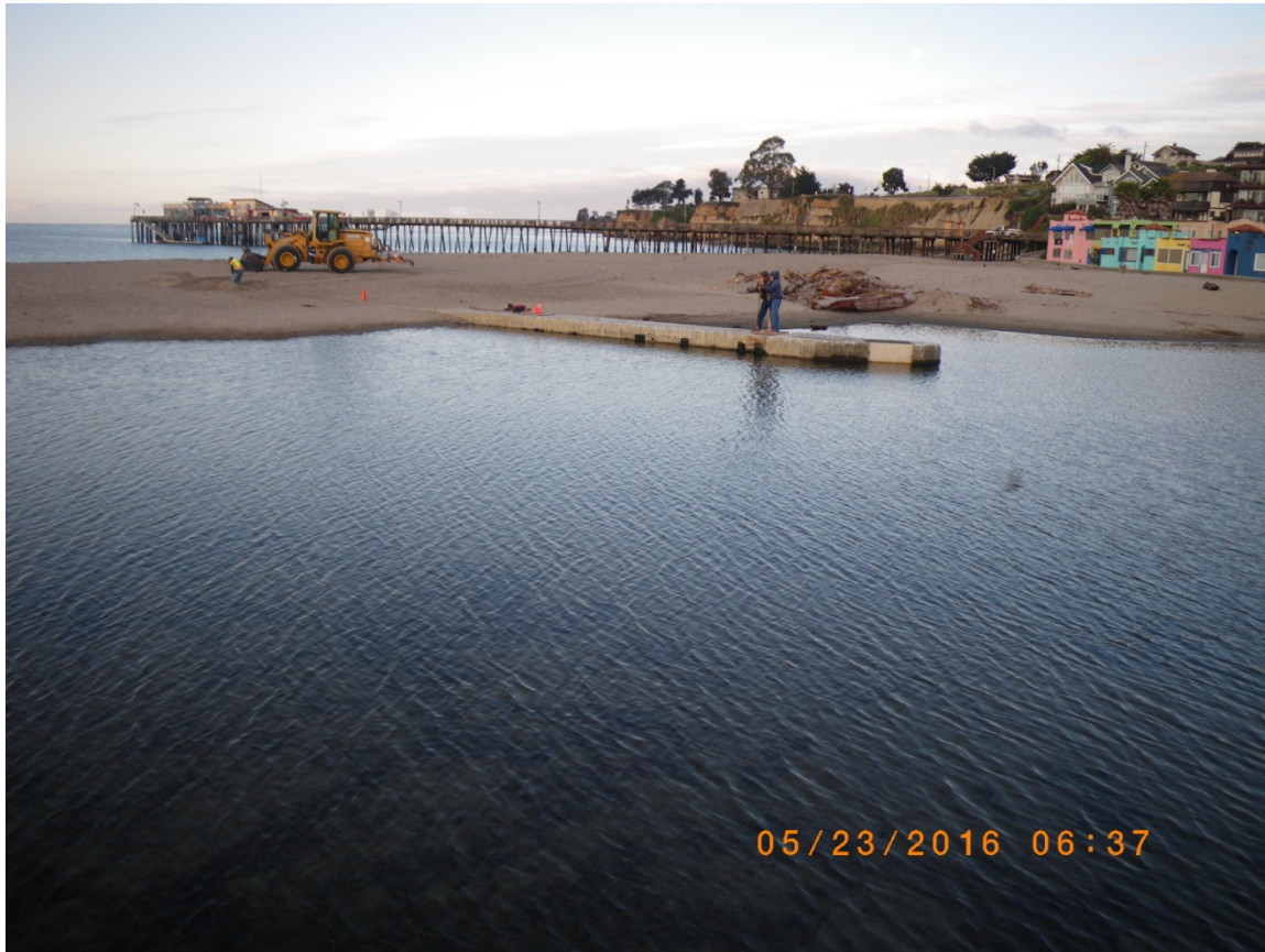
Soquel Estuary and flume inlet before construction activities began.
