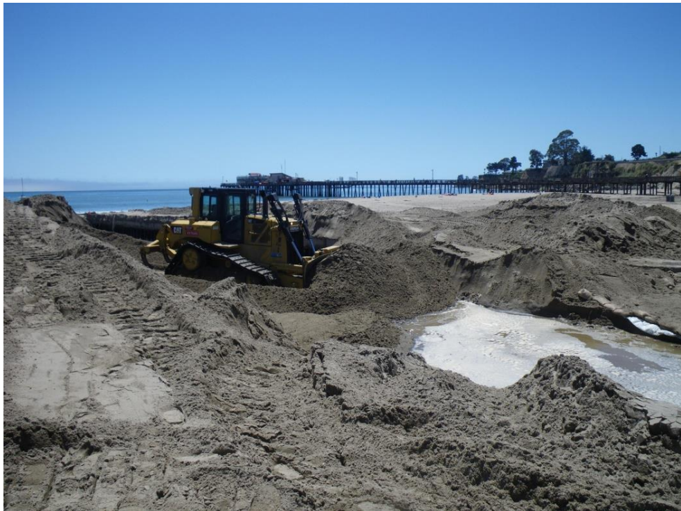
Final closure of sandbar outlet channel for summer season. 1 June 2017; 1335 hr.
