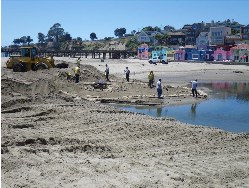
Completion of flume inlet preparation prior to final sandbar closure. 1 June 2017
