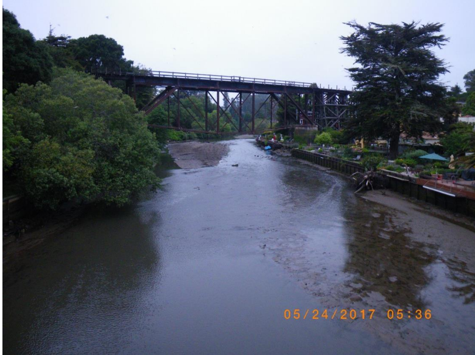
Estuary upstream of Stockton Bridge resulting from unplanned sandbar breach. (Add 1 hour to time stamp.) 24 May 2017
