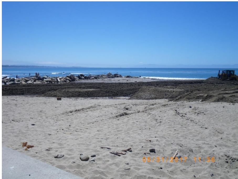
Sand being stockpiled at a low point along the jetty. 31 May 2017
