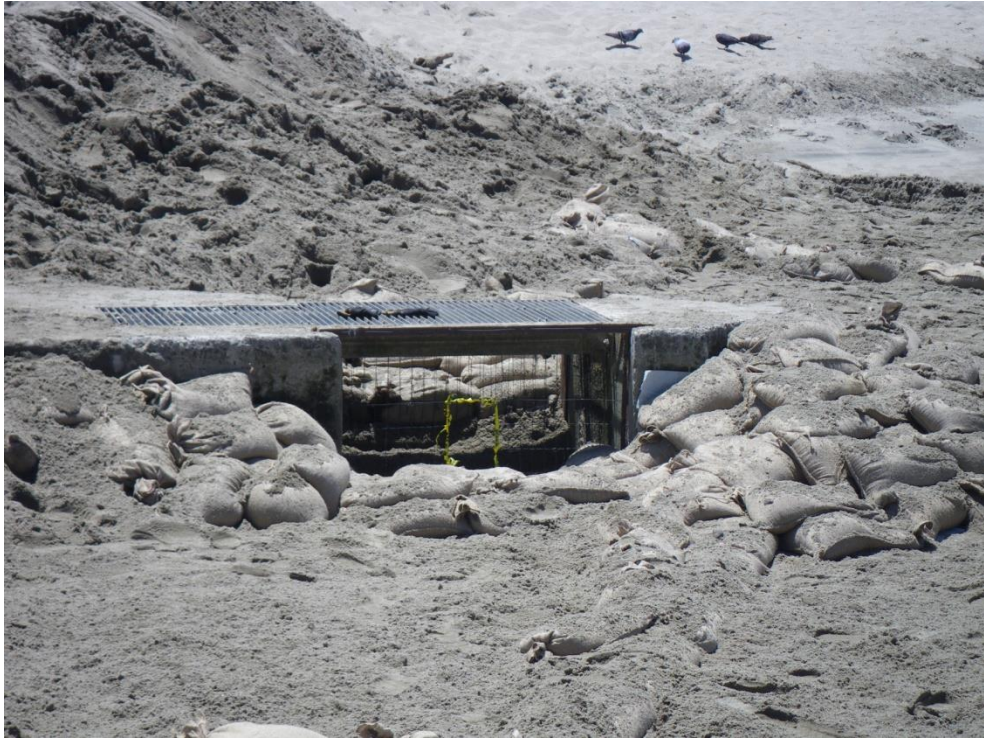
Underwater portal provided for adult salmonid passage through flume. 1 June 2017
