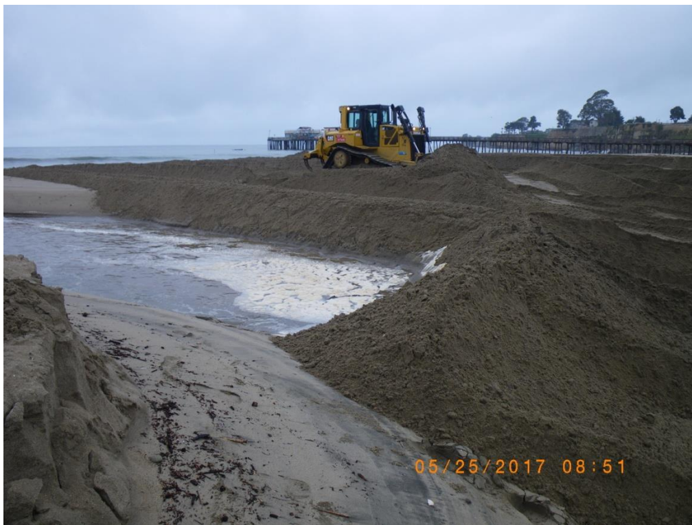
Outlet channel closed off to create the temporary lagoon prior to Memorial Day weekend. 25 May 2017
