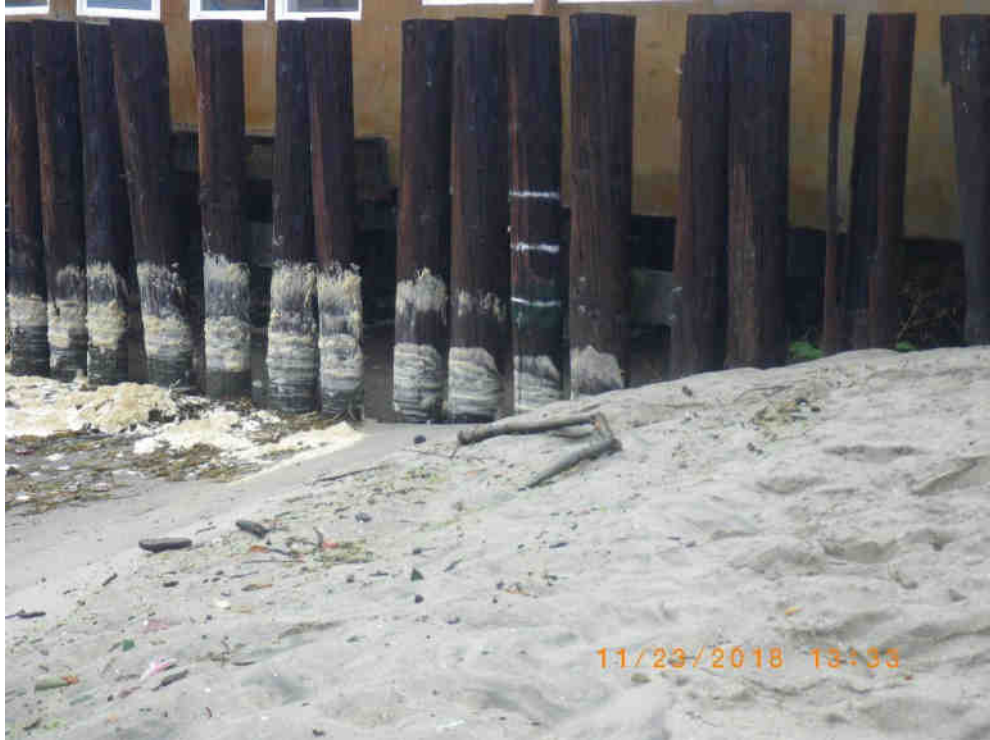
Estuary Water Surface in Relation to lower piling ring with bent bolt midday after sandbar breach. 23 November 2018
