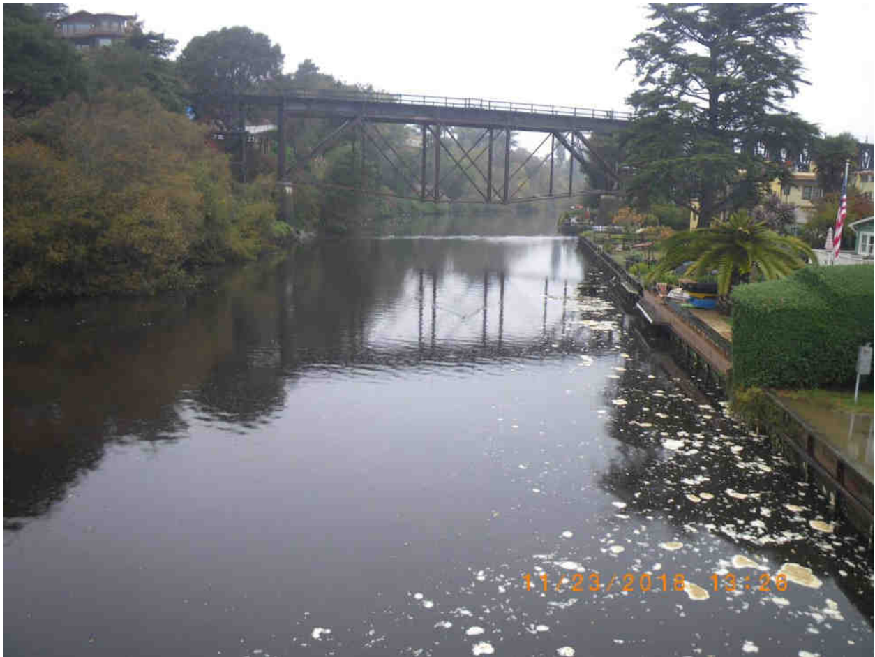
View of the estuary, looking upstream from Stockton Bridge at midday after sandbar breach. 23 November 2018
