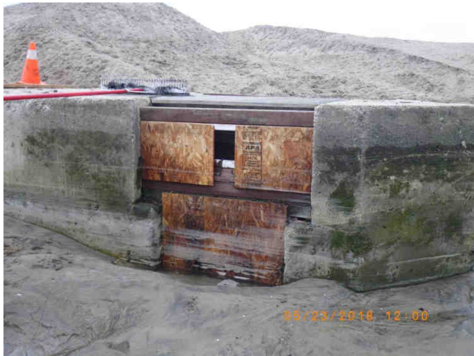
Flume underwater portal prepared for sandbar closure 23 May 2018
