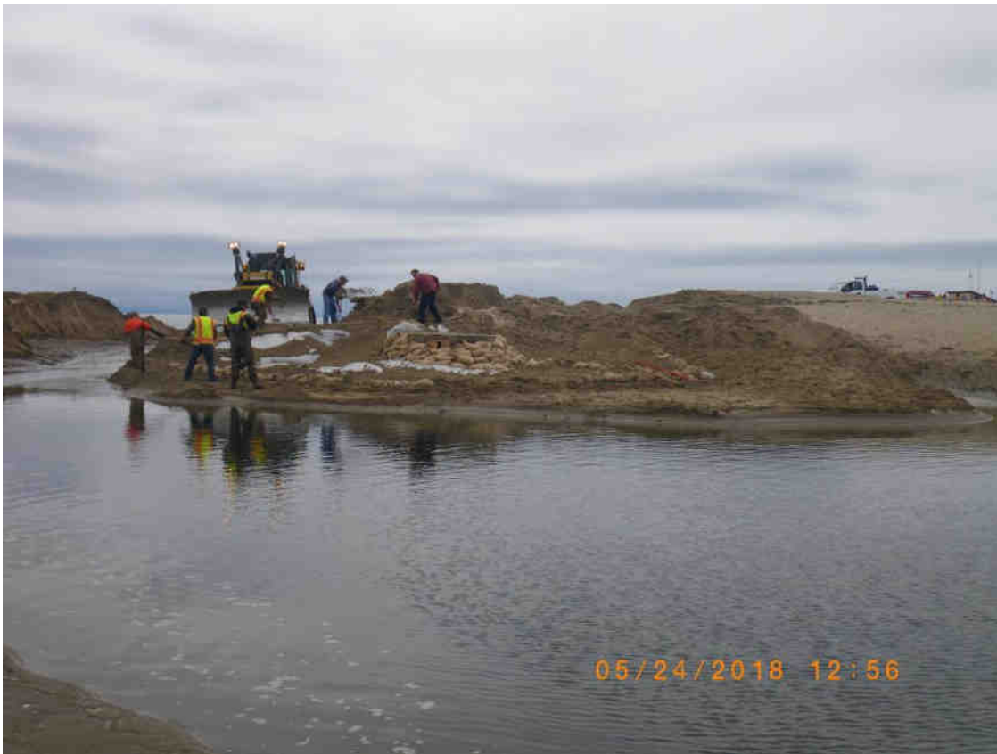
Flume inlet preparation prior to final sandbar closure for summer. 24 May 2018
