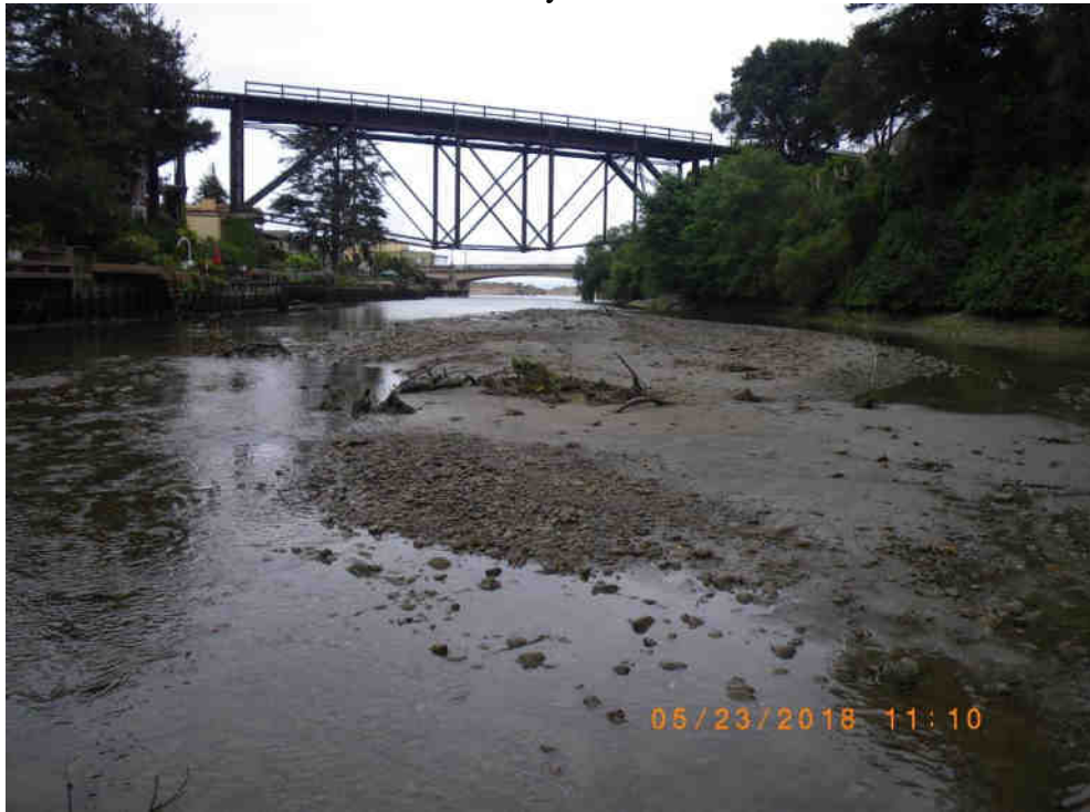
Estuary looking downstream at mid-channel bar above trestle (no stranded fish). 23 May 2018
