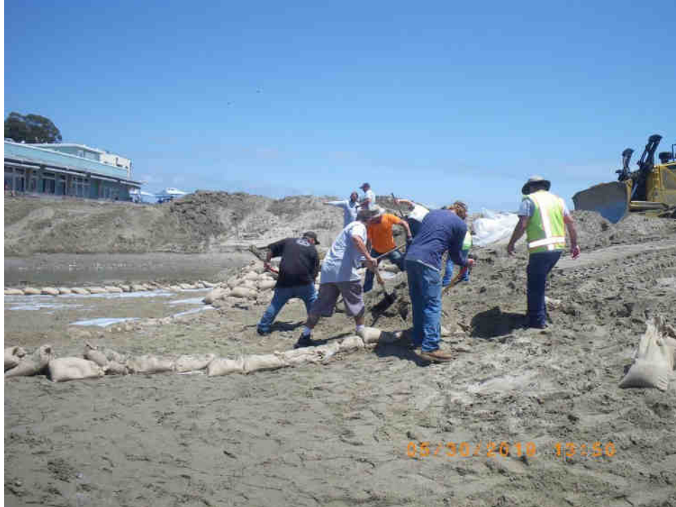
Public Works Staff covering the visquine with sand. 30 May 2019
