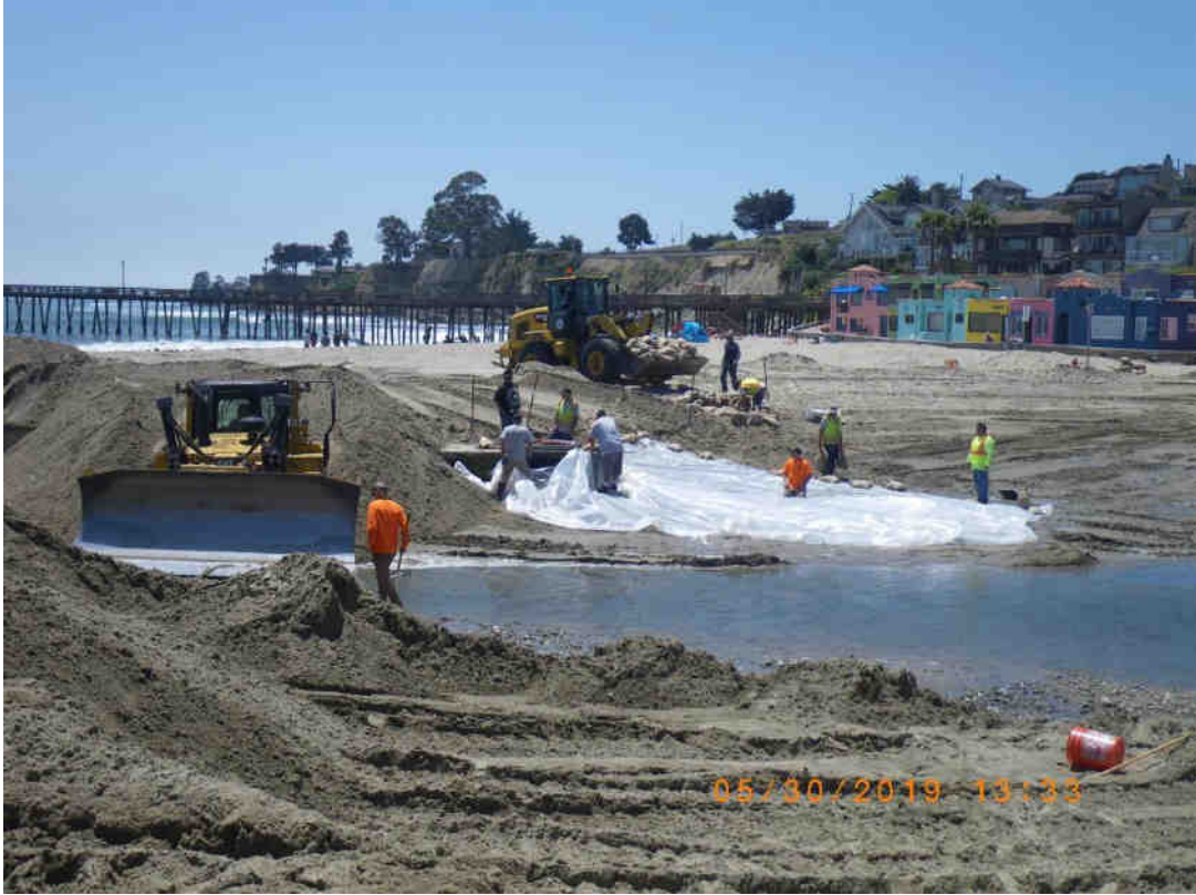
Visquine being spread over the flume inlet pad. 30 May 2019
