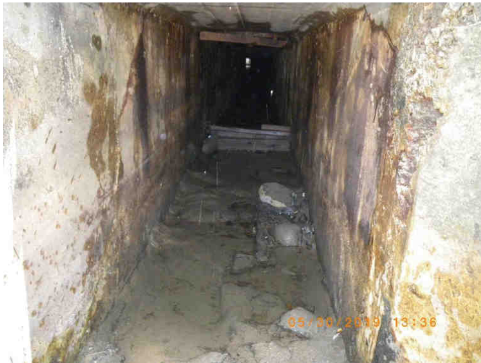
Weir intact inside the flume. 30 May 2019
