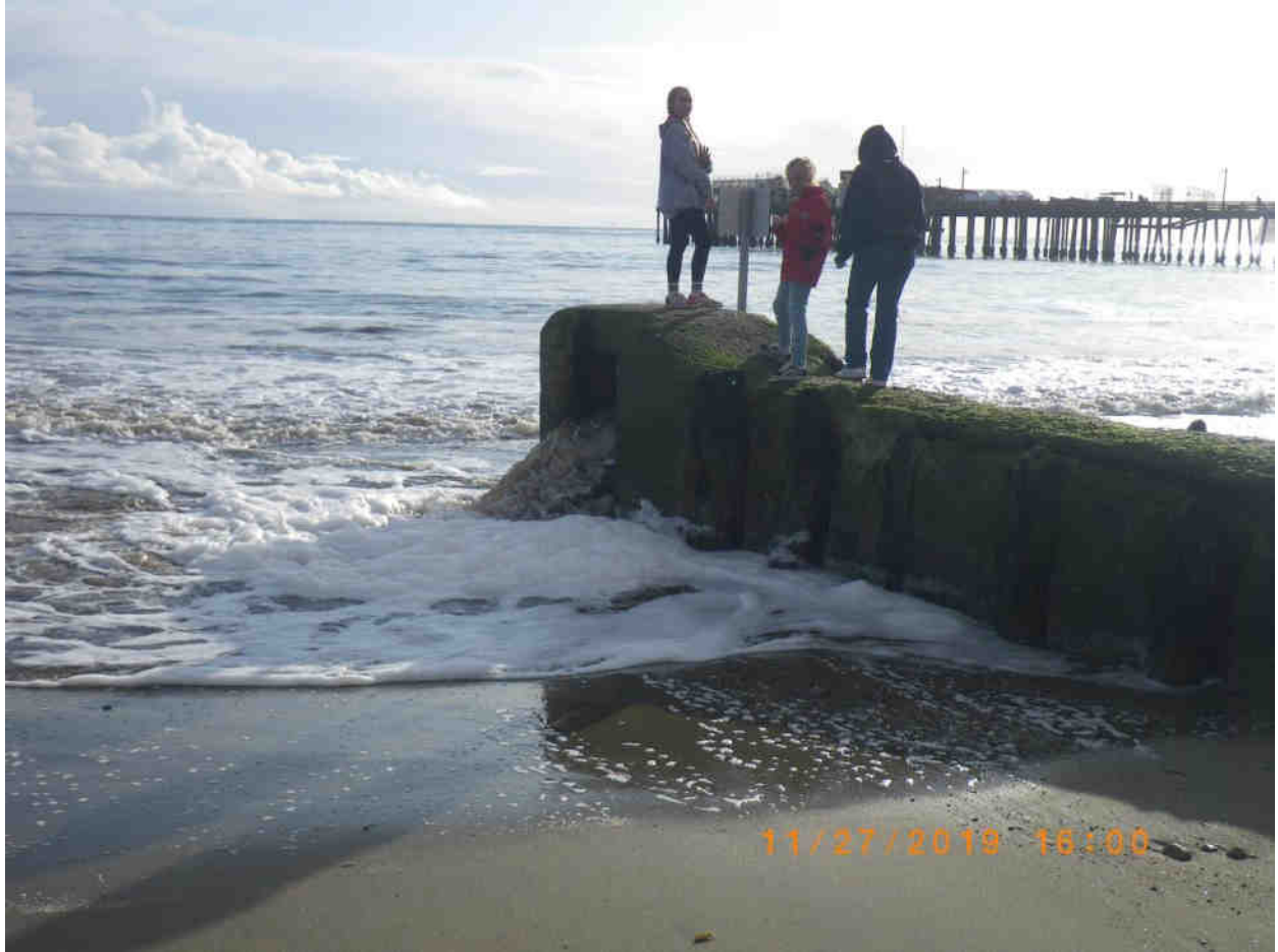
Flume outlet conveying water and maintaining water transfer through lagoon during low tide. 27 November 2019
