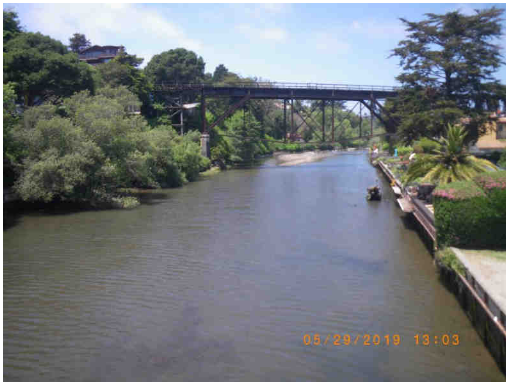
Estuary looking upstream from Stockton Bridge at maximum estuary drawdown. 29 May 2019
