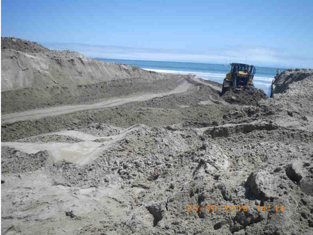
Kotila packing sand under the flume during sandbar closure. 30 May 2019
