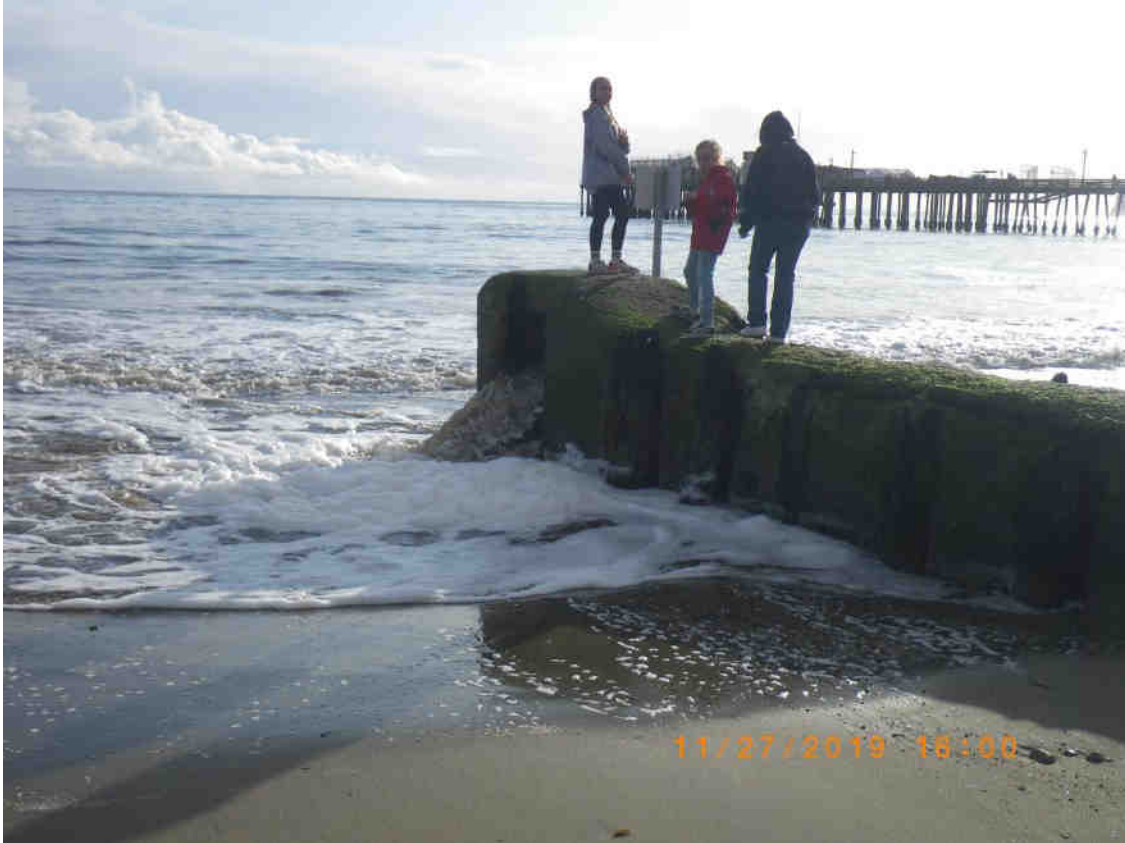
Flume outlet conveying lagoon water and maintaining water transfer through lagoon during low tide. 27 November 2019
