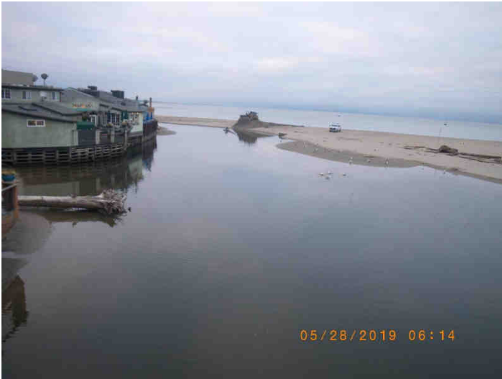
Soquel Estuary prior to sandbar construction.
