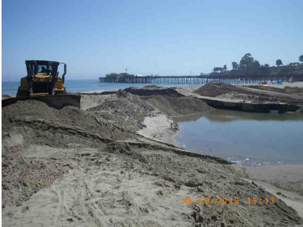
Kotila building the berm around the lagoon periphery.
