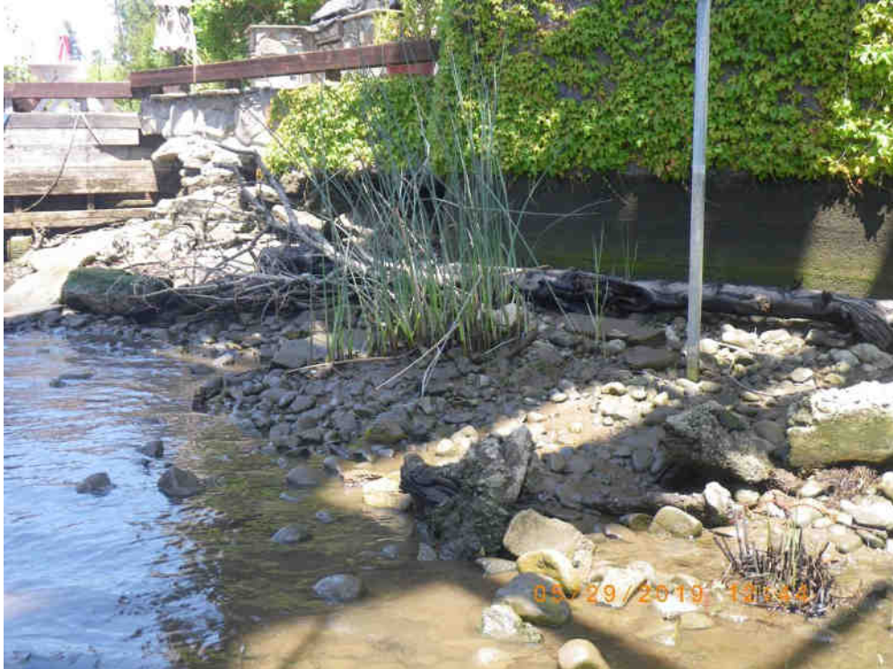
Cattails survived the wet winter in the railroad trestle cove. 29 May 2019
