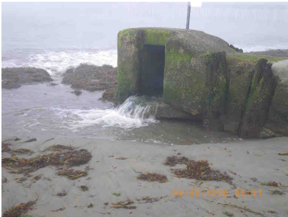
Flume outlet to the Monterey Bay. 22 August 2020
