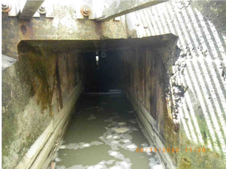
Weir inside flume intact, creating a pool for fish at inlet. 11 June 2020
