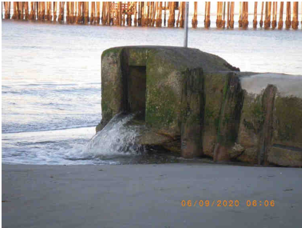
Streamflow passing through the flume overnight to provide steelhead smolt passage. 9 June 2020
