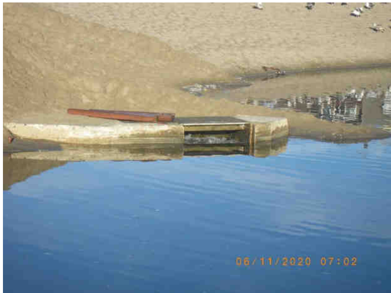
Lagoon filled overnight, and 2 boards were removed at 0630 hr to reduce the head of water when the sandbar was opened 11 June 2020
