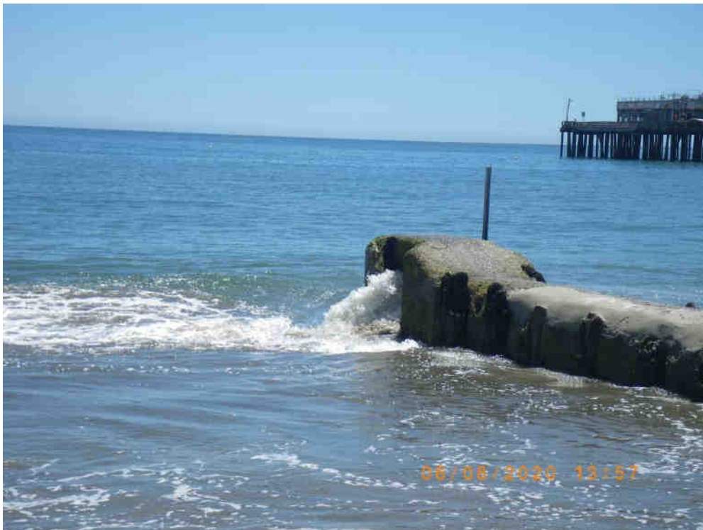
Flume cleared of sand with its first flush of streamflow from the lagoon that had overtopped the flume before clearance. 8 June 2020
