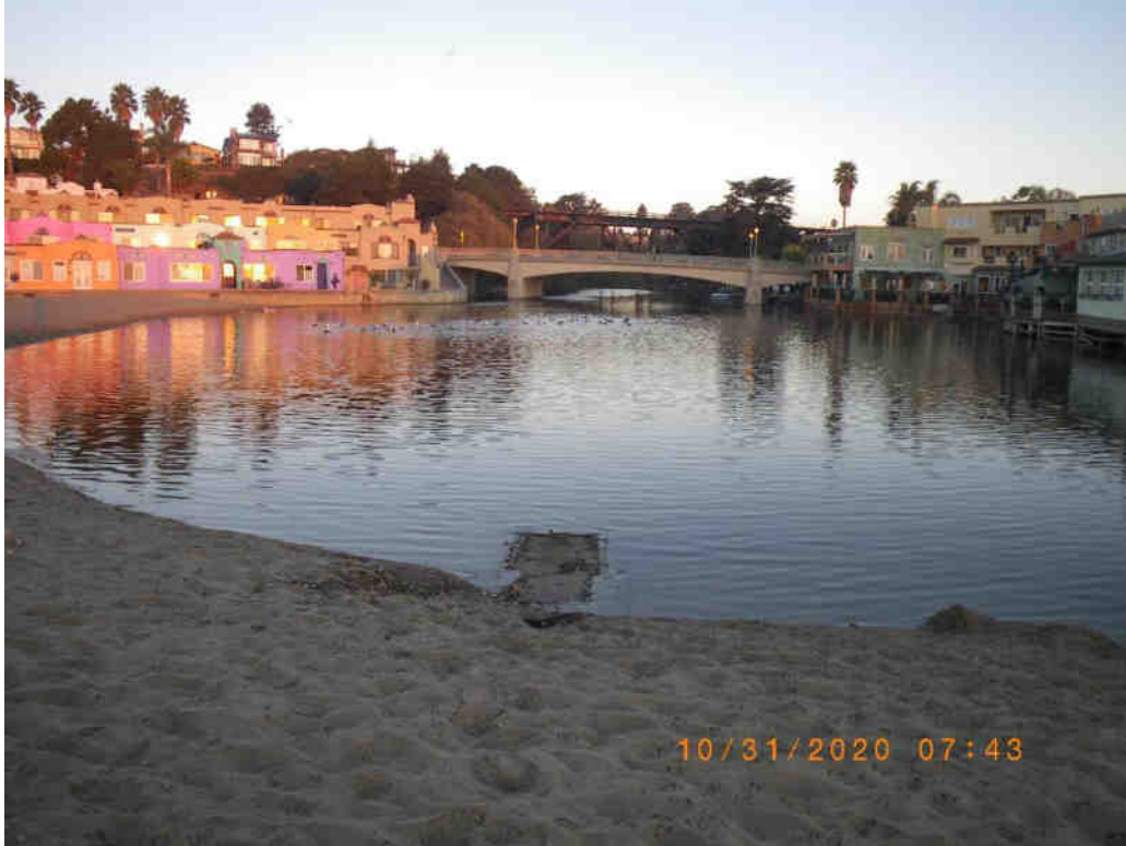
Reach 1, looking upstream from the flume inlet (foreground) –Venetian Court on the left; Esplanade restaurants and Margaritaville Cove on the right; Stockton Bridge in center. 31 October 2020
