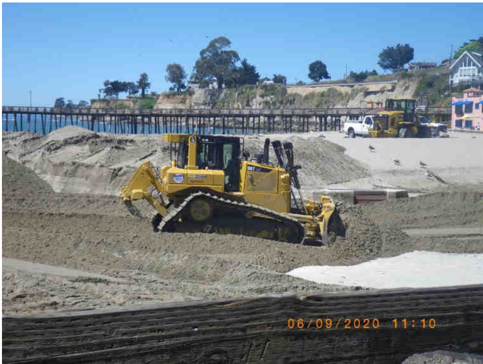
Kotila contouring around the flume inlet after sandbar closure. 9 June 2020
