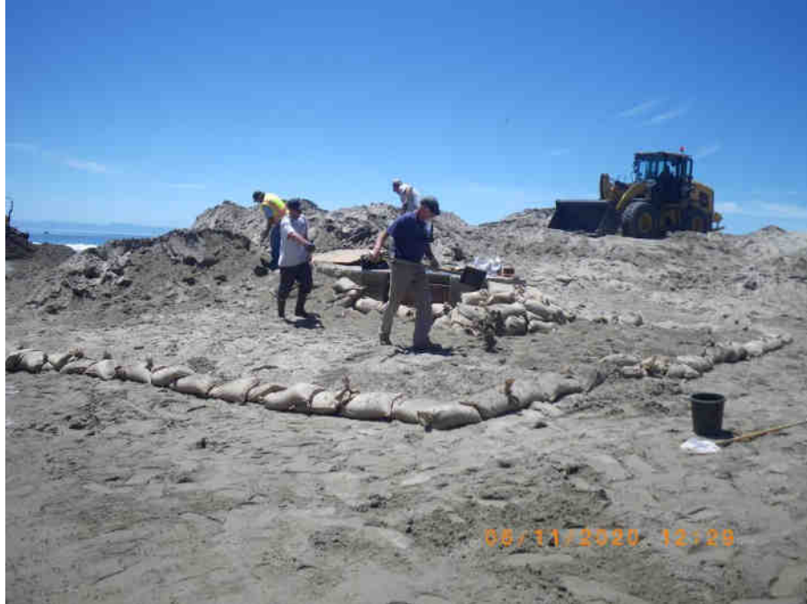
Visquine covered with sand by hand shovel, with sandbags around the flume inlet. 11 June 2020
