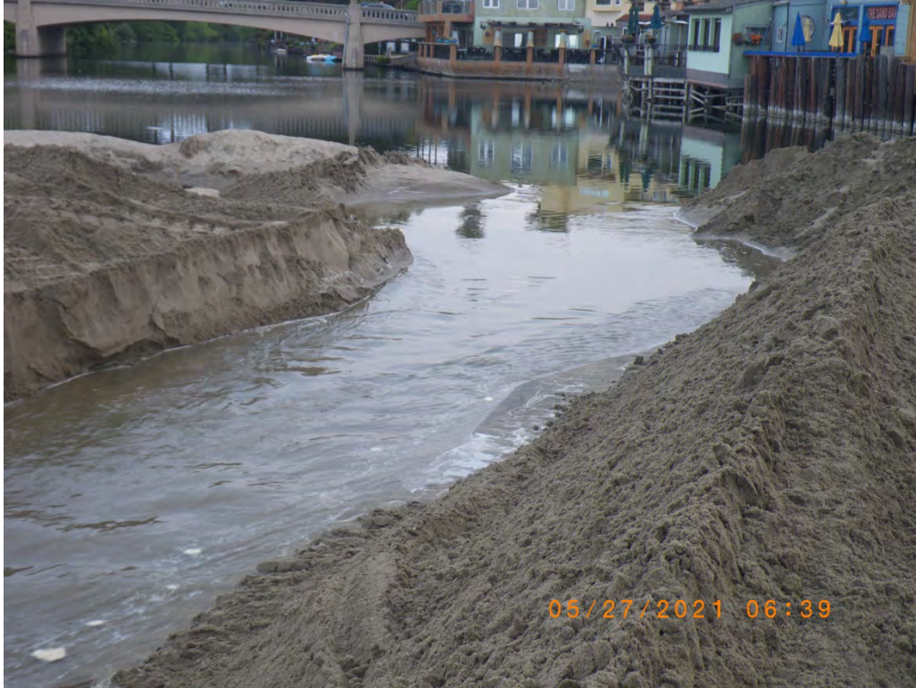
Outlet channel. 27 May 2021
