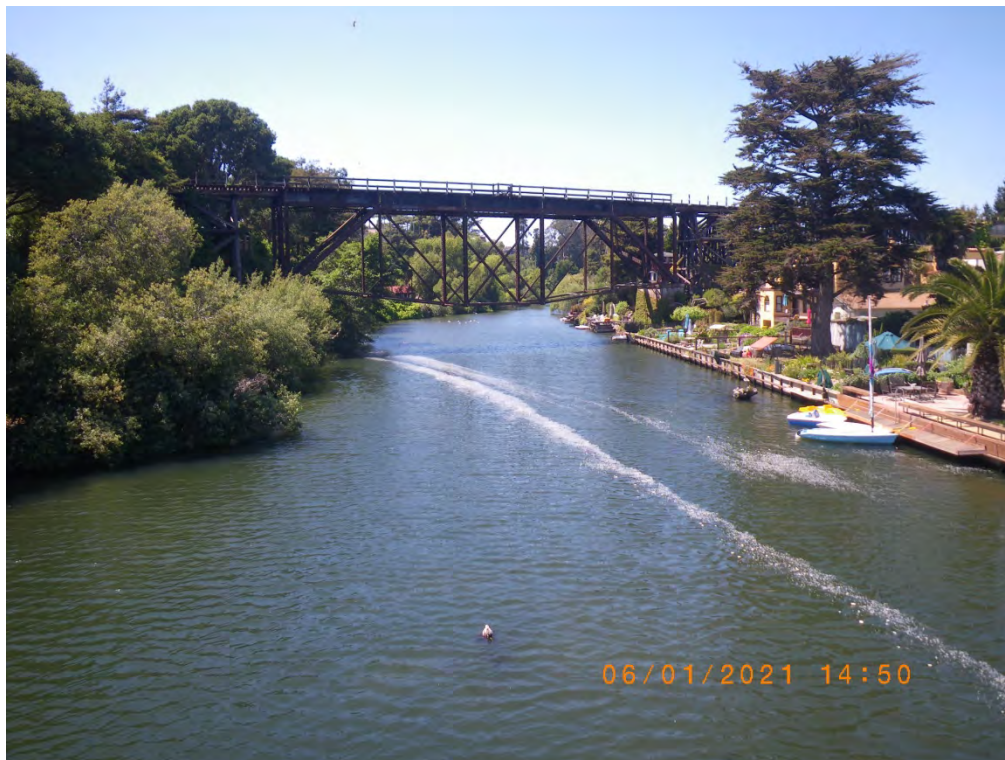
Upper lagoon after sandbar closure and flume preparation. 1 June 2021
