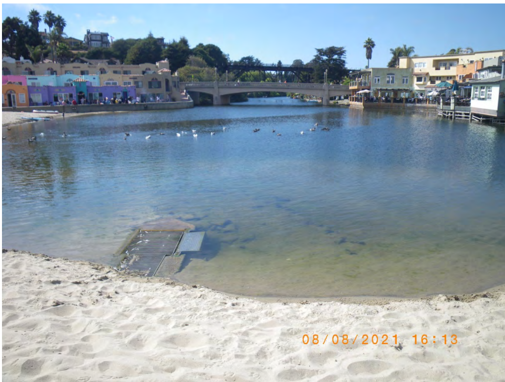
Reach 1- Looking upstream with flume inlet in foreground and Venetian Court on left. 8 August 2021
