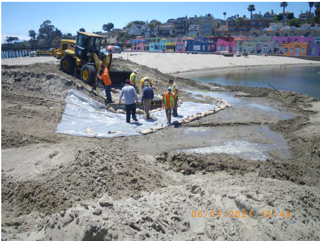
Visquine sheeting spread out and secured around the flume inlet. 1 June 2021
