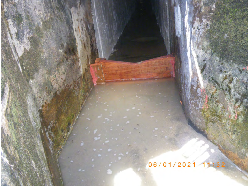
Interior weir installed in flume, upstream of fiberglassed section. 1 June 2021
