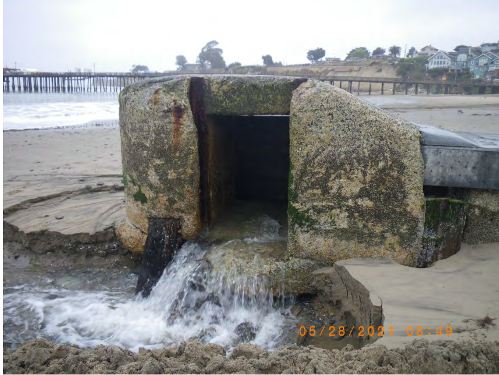
Flume outfall. 28 May 2021
