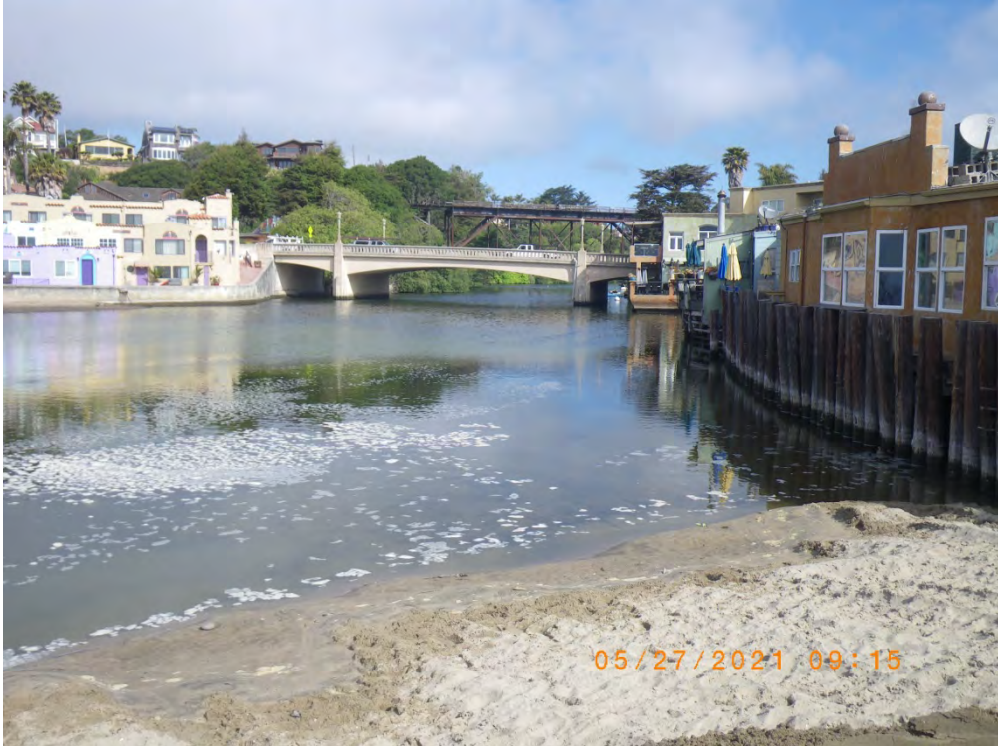
Receded lagoon margin immediately after sandbar closure. 27 May 2021
