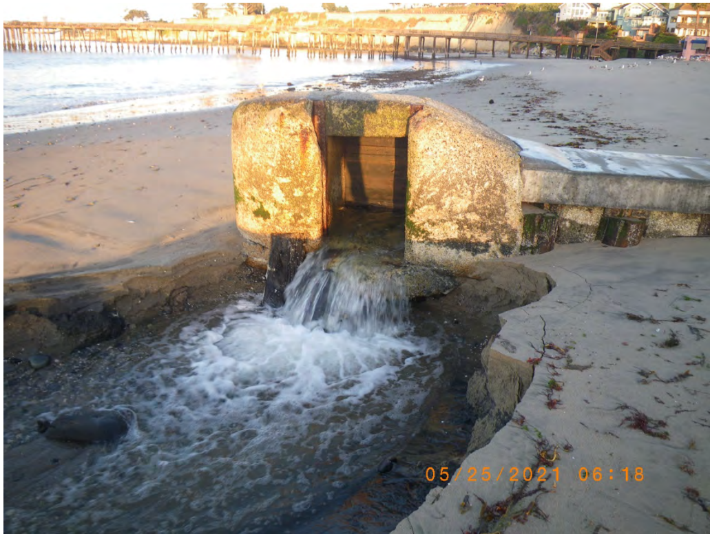
Streamflow passing through the flume the previous night for smolt passage. 25 May 2021
