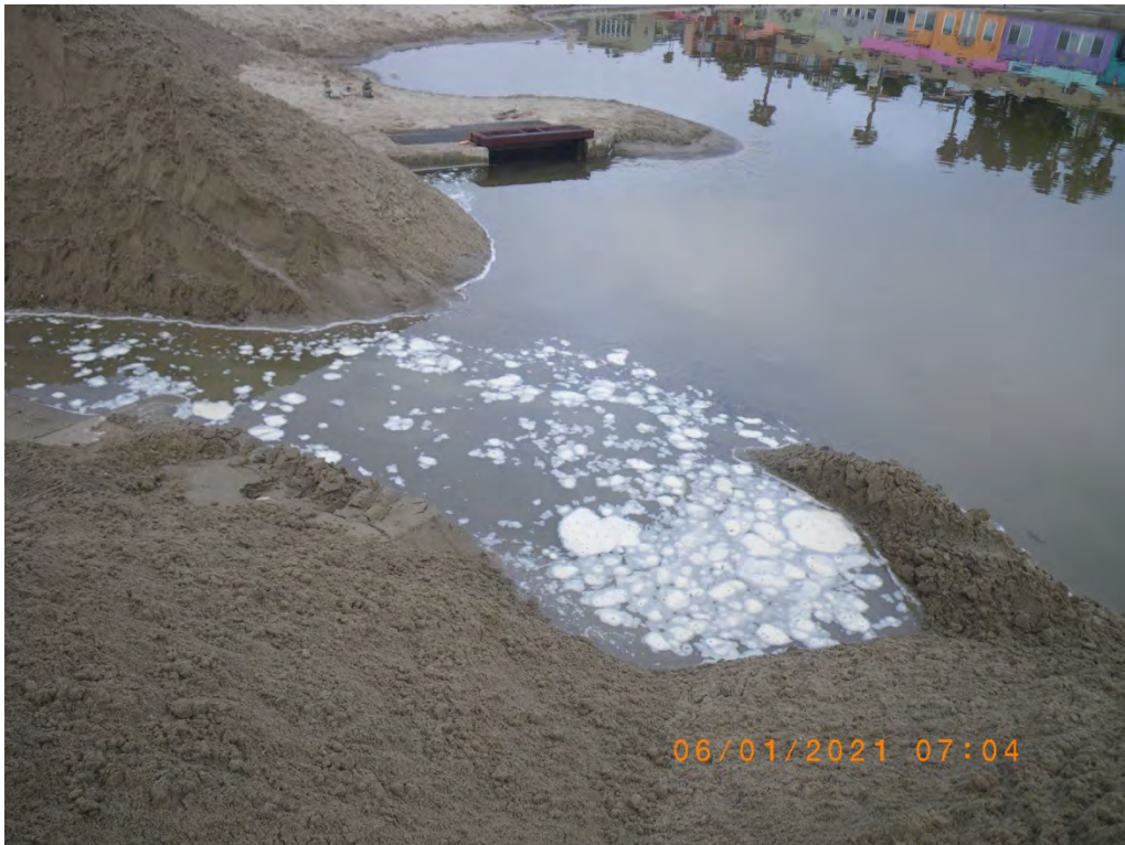
Outlet channel cut adjacent to the flume inlet. 6-01-2021
