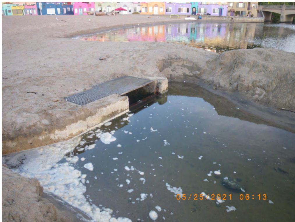
Lagoon spilling over flashboards with smolt passage previous night. 25 May 2021
