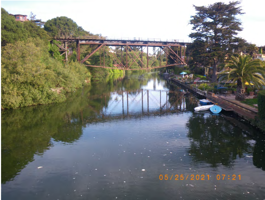
Upper lagoon viewed from Stockton Bridge upstream. 25 May 2021
