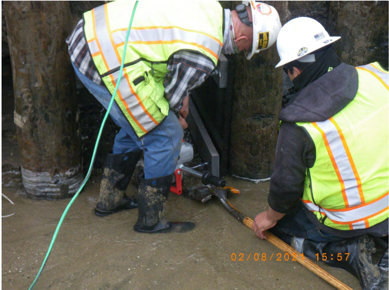
Cut-off wall being secured to pilings under the flume. 8 February 2021
