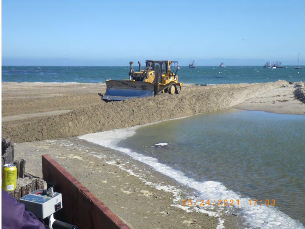
Kotila covering the lateral channel after fish relocation. 24 May 2021
