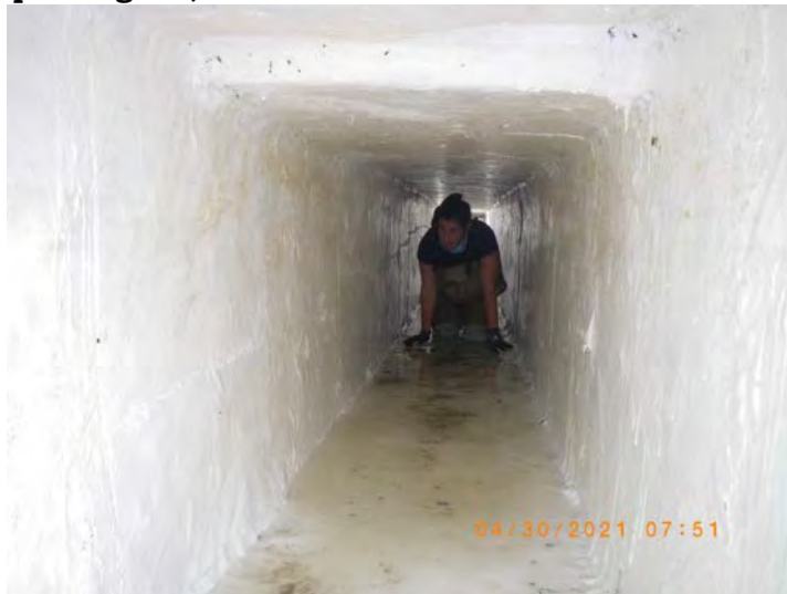
Flume Interior during Final Inspection after Rehabilitation, April 2021
