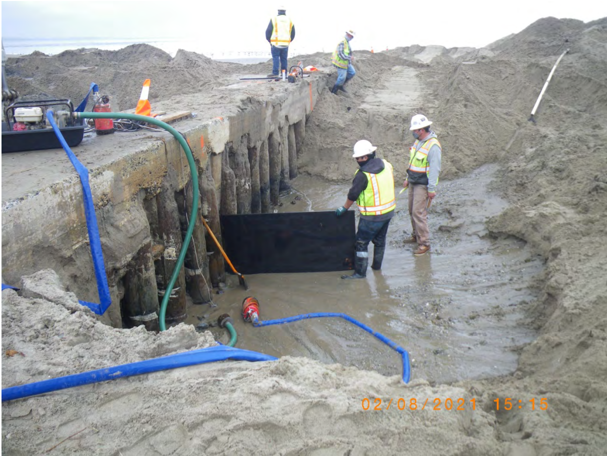
Cut-off wall to be secured under the flume. 8 February 2021
