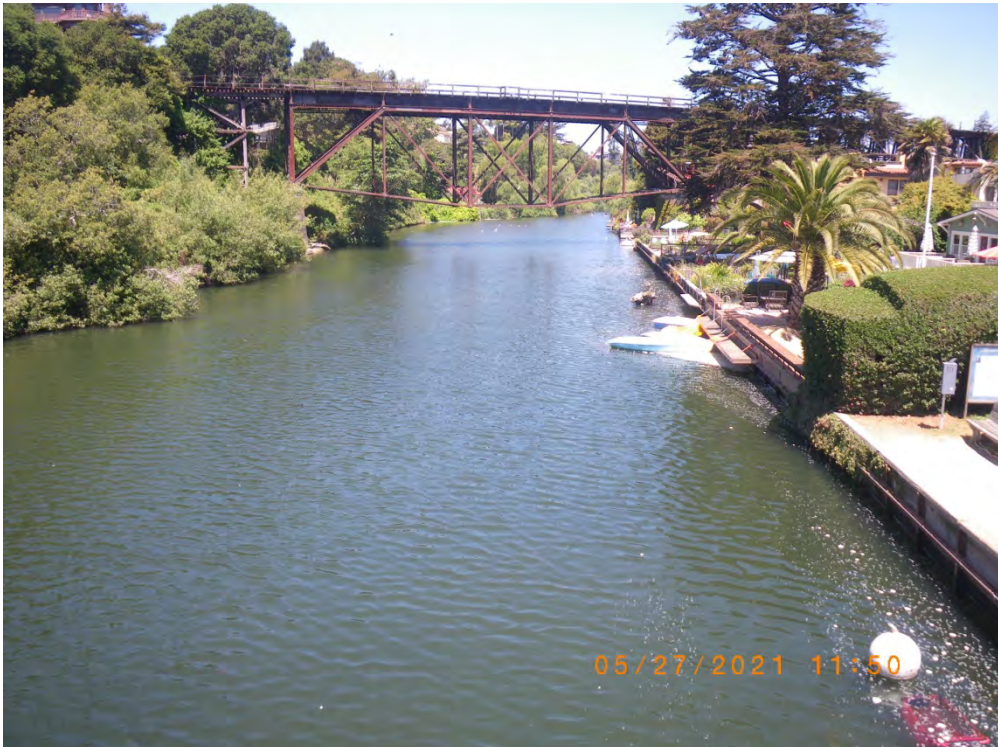
Lagoon width maintained upstream of Stockton Bridge during flume preparation. 27 May 2021
