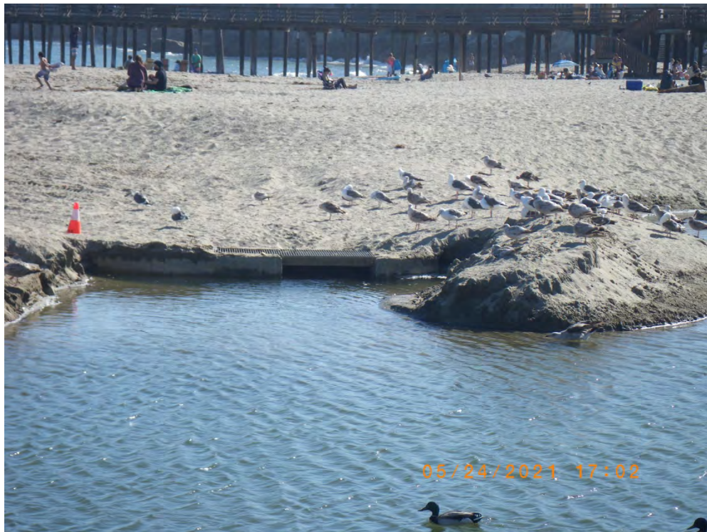
Steelhead passage provided through the flume by the end of the day. 24 May 2021
