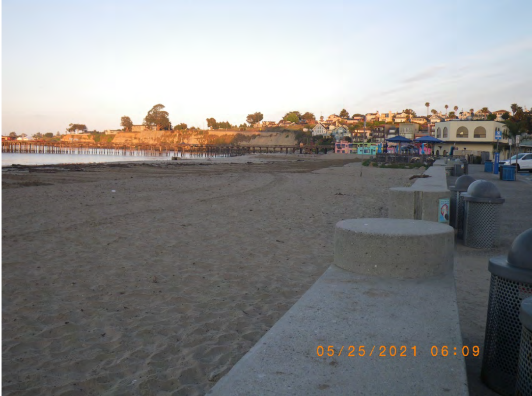
Lateral channel conversion to beach completed the previous day. 25 May 2021
