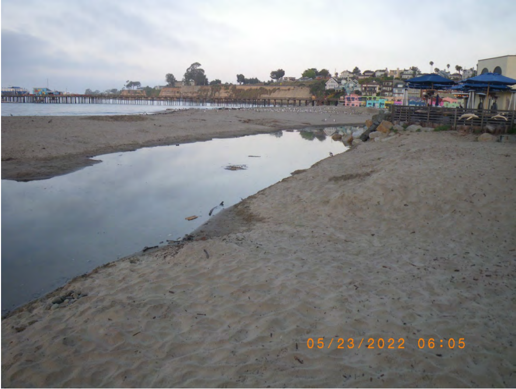
Lateral channel ponded diagonally across the beach, looking upstream toward the flume. 23 May 2022
