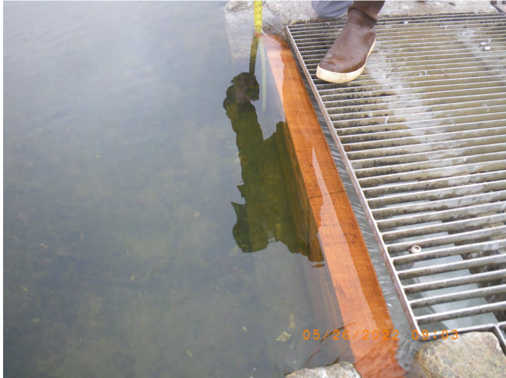
Lagoon filled overnight with added flashboards, providing smolt steelhead passage the previous night. 26 May 2022
