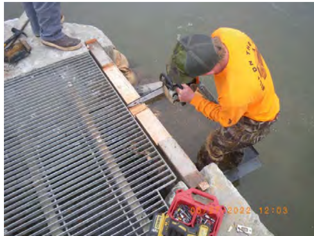
Sanden Notching the Uppermost Flashboard (Flume Inlet) for Steelhead Smolt Passage, May 2022
