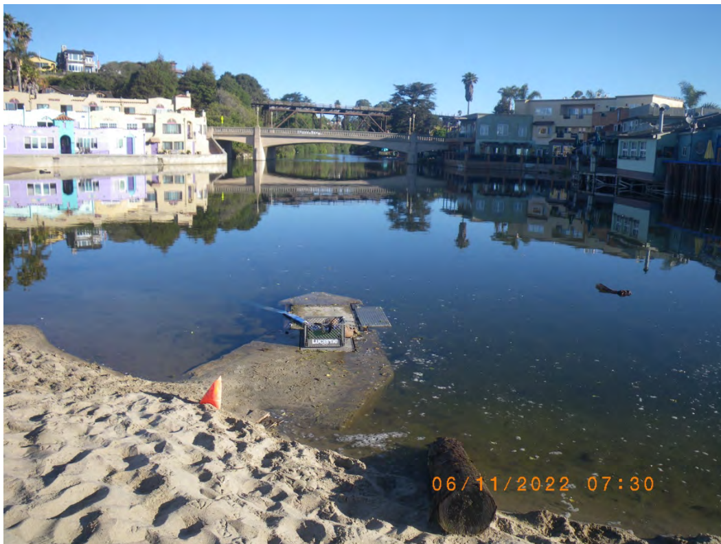
Reach 1- Looking upstream with flume inlet in foreground and Venetian Court on left. 11 June 2022
