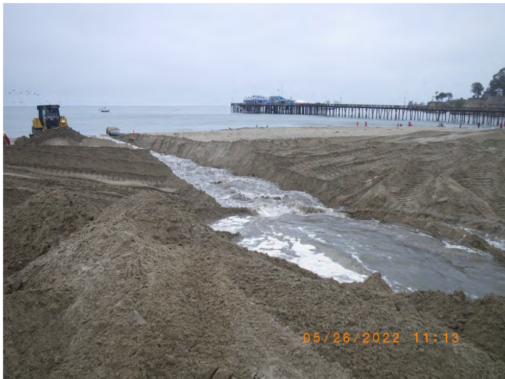
Outlet channel with slow lagoon drawdown. 26 May 2022
