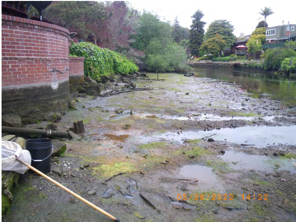
Receded lagoon adjacent to the Shadowbrook Restaurant wall, looking upstream. 26 May 2022
