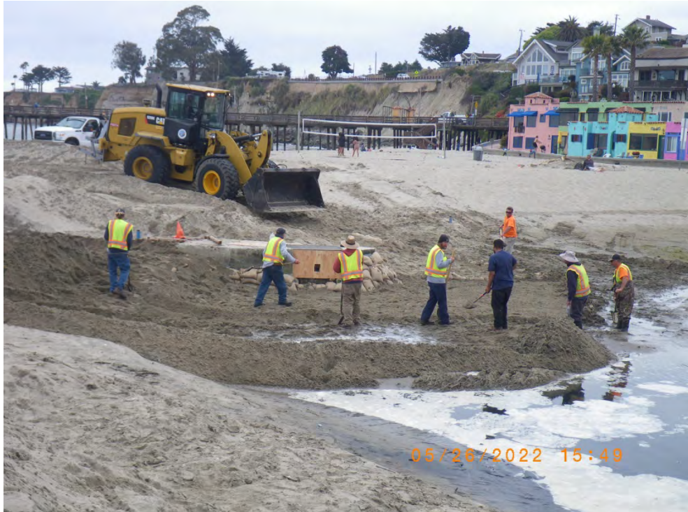
Public Works staff covering visquine sheet with sand. 26 May 2022
