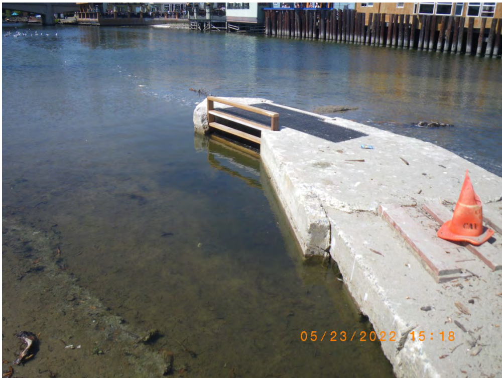
Steelhead passage provided through the wooden frame and flume inlet at the end of the day. 23 May 2022
