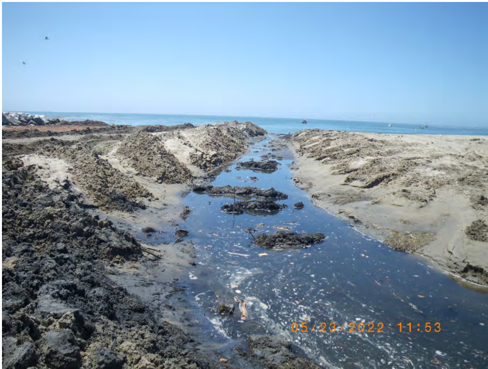
Sandbar opened near the jetty to partially drain the lateral channel. 23 May 2022
