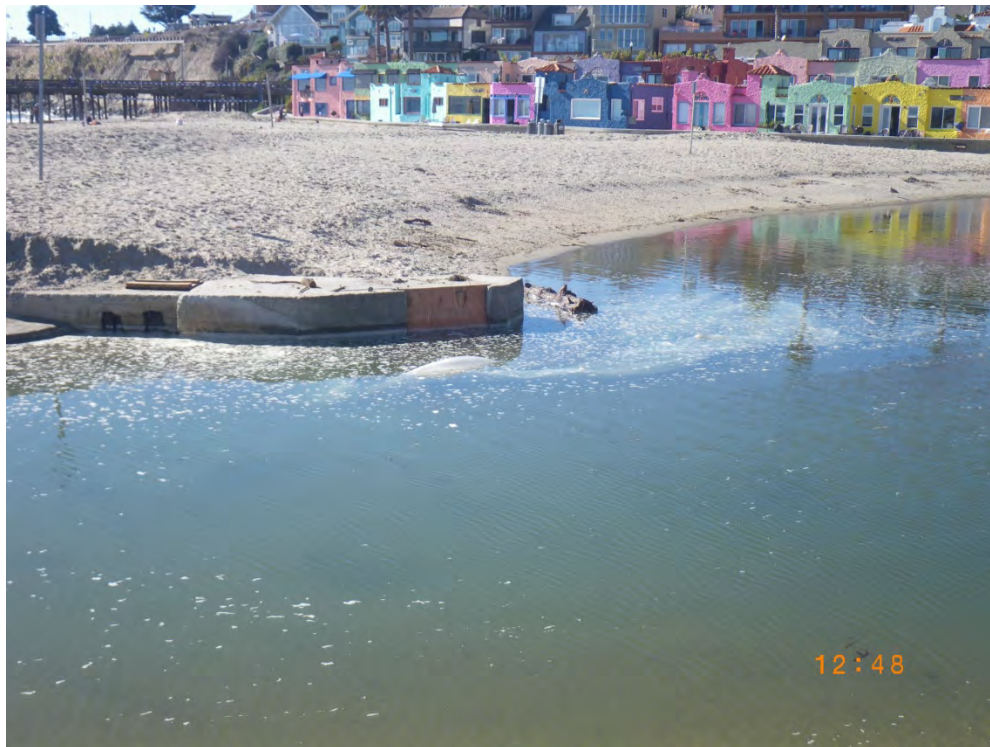
Flume inlet sealed for the winter. at 1.7 cfs at Soquel Village gage. 1248 hr, 13 November 2022.
