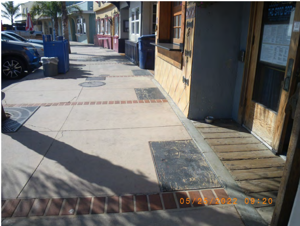
Covered Esplanade sidewalk drains. 25 May 2022
