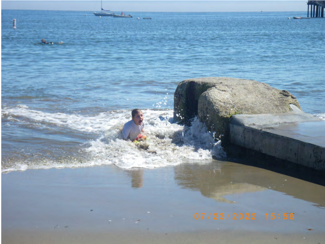
Flume outlet to the Capitola Beach and Monterey Bay. 23 July 2022
