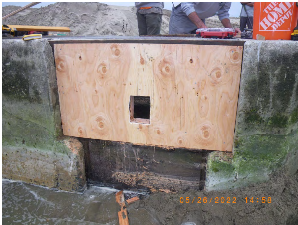
Underwater adult steelhead portal completed on the flume inlet, restaurant side. 26 May 2022
