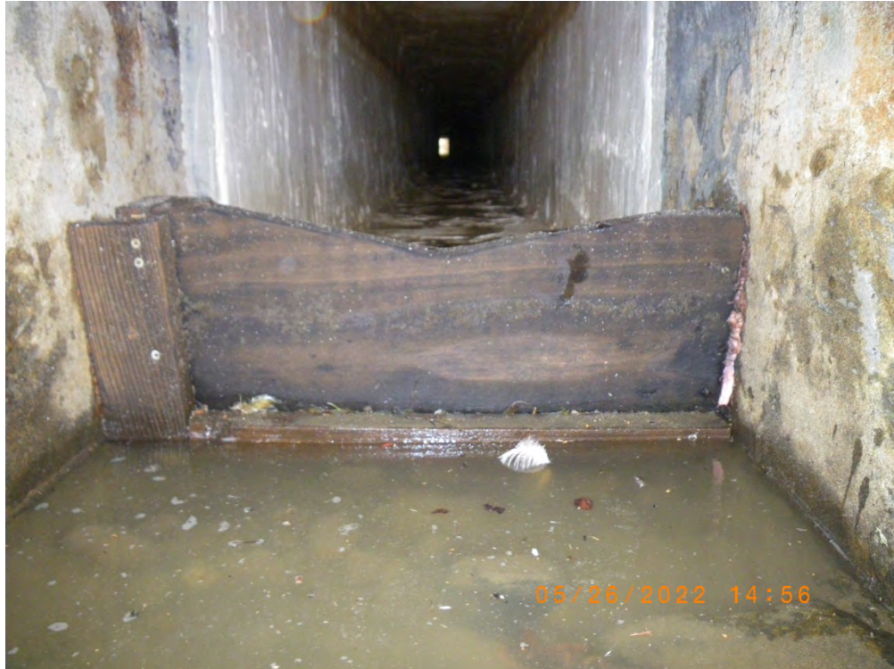
Weir intact inside the flume. New lining visible. 26 May 2022
