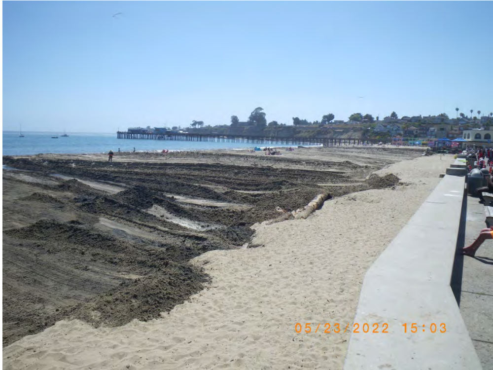
Lateral channel covered with sand after fish relocation. 23 May 2022
