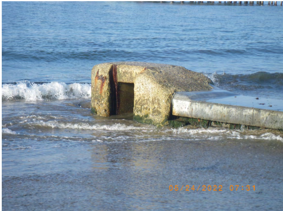
Streamflow passing through the flume the previous night for smolt passage. 24 May 2022
