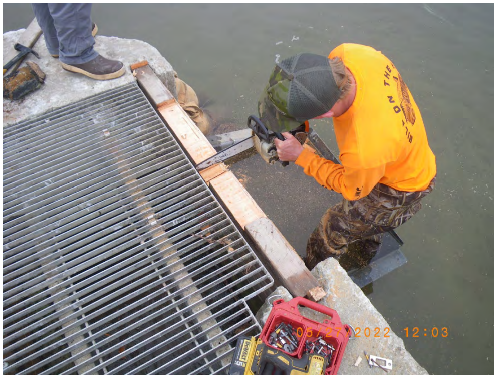
Cooper Sanden notching the upper flashboard for steelhead smolt passage. 27 May 2022
