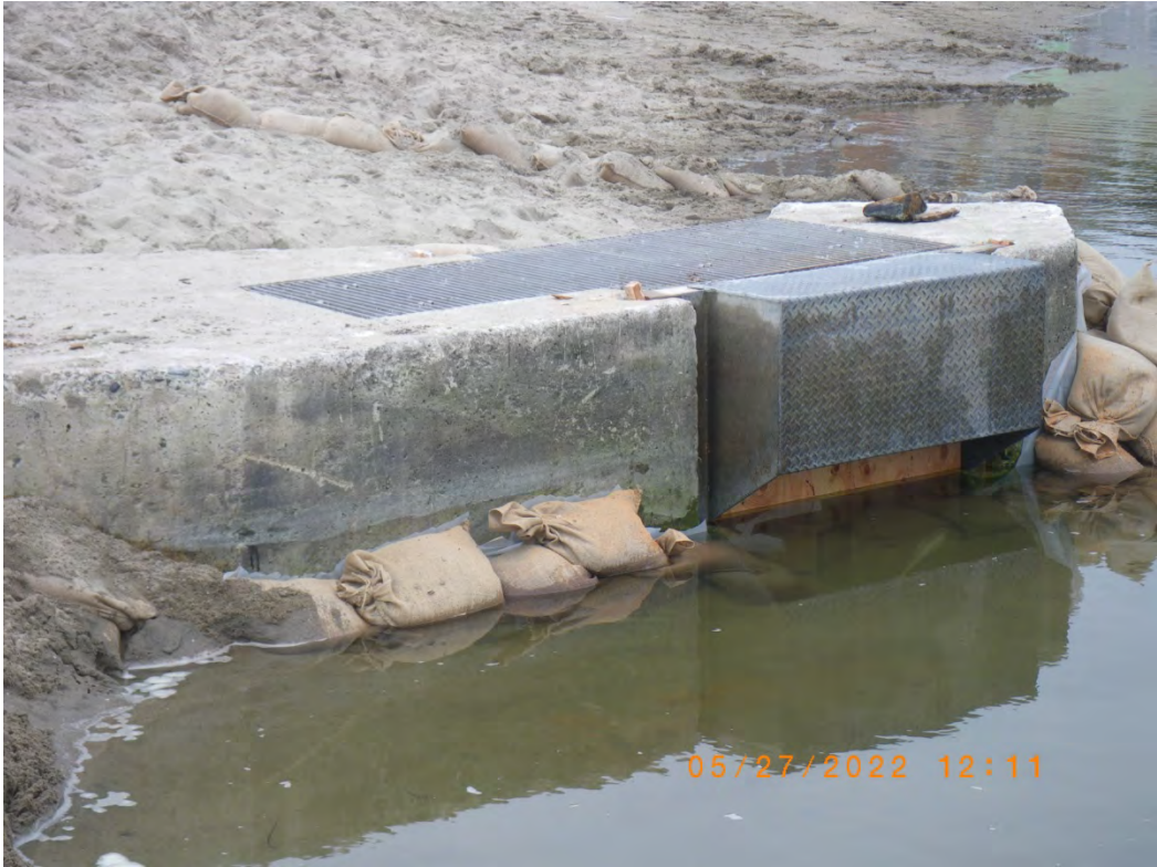
Shroud attached to flume inlet. 27 May 2022
