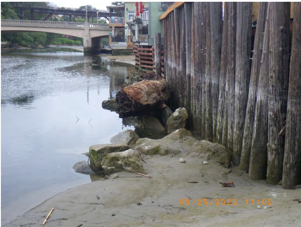
Entrained redwood log adjacent to restaurant pilings. 25 May 2023
