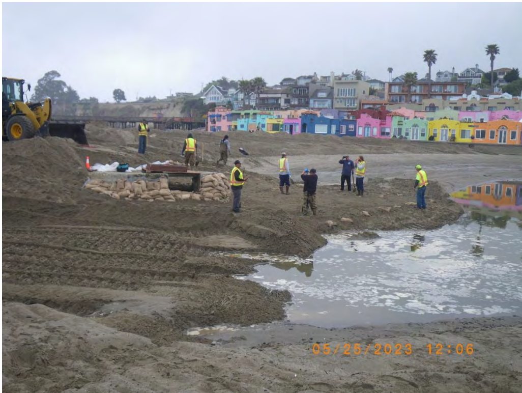
Pad completed around flume inlet. 25 May 2023
