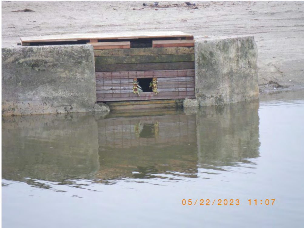
Steelhead passage provided through the flume inlet. 22 May 2023
