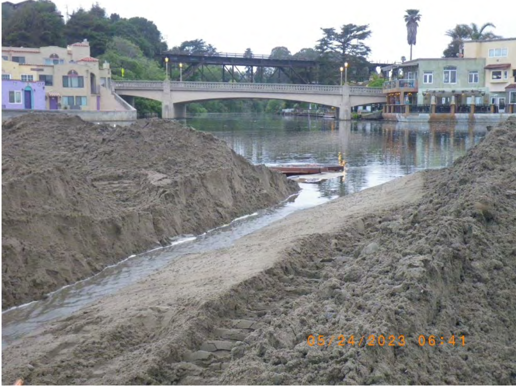
Outlet channel cut through sandbar next to the flume. 24 May 2023
