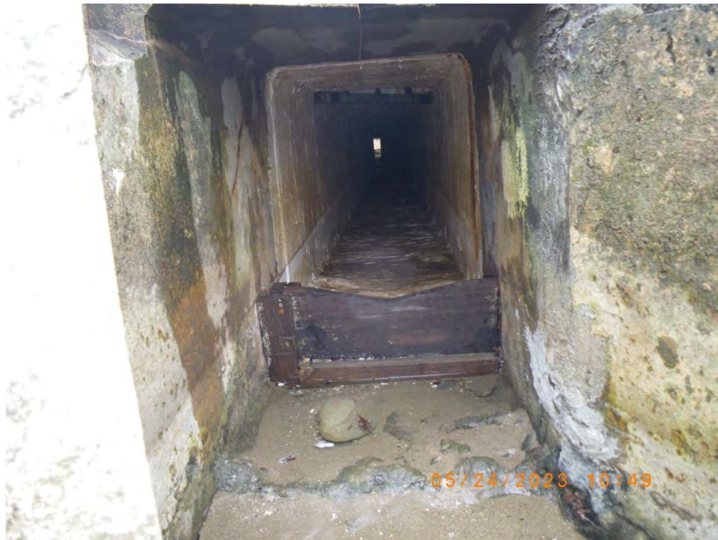
Intact weir inside the flume near the inlet. 24 May 2023
