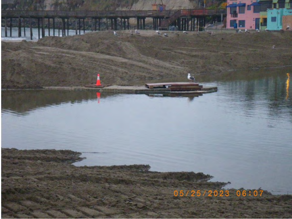
Flume inlet with screens pulled in early morning. Lagoon filled overnight. 25 May 2023
