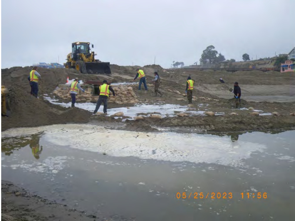
Public Works staff covering visquine with sand at flume inlet. 25 May 2023
