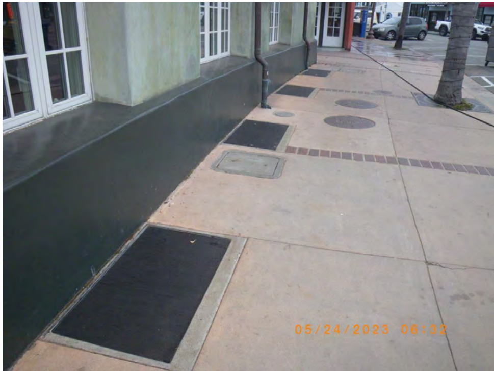
Sidewalk drains covered. 24 May 2023
