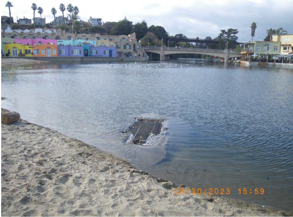
Reach 1- Flume inlet with Venetian Court on left, Stockton Bridge in center and Margaritaville Cove on right. 30 September 2023
