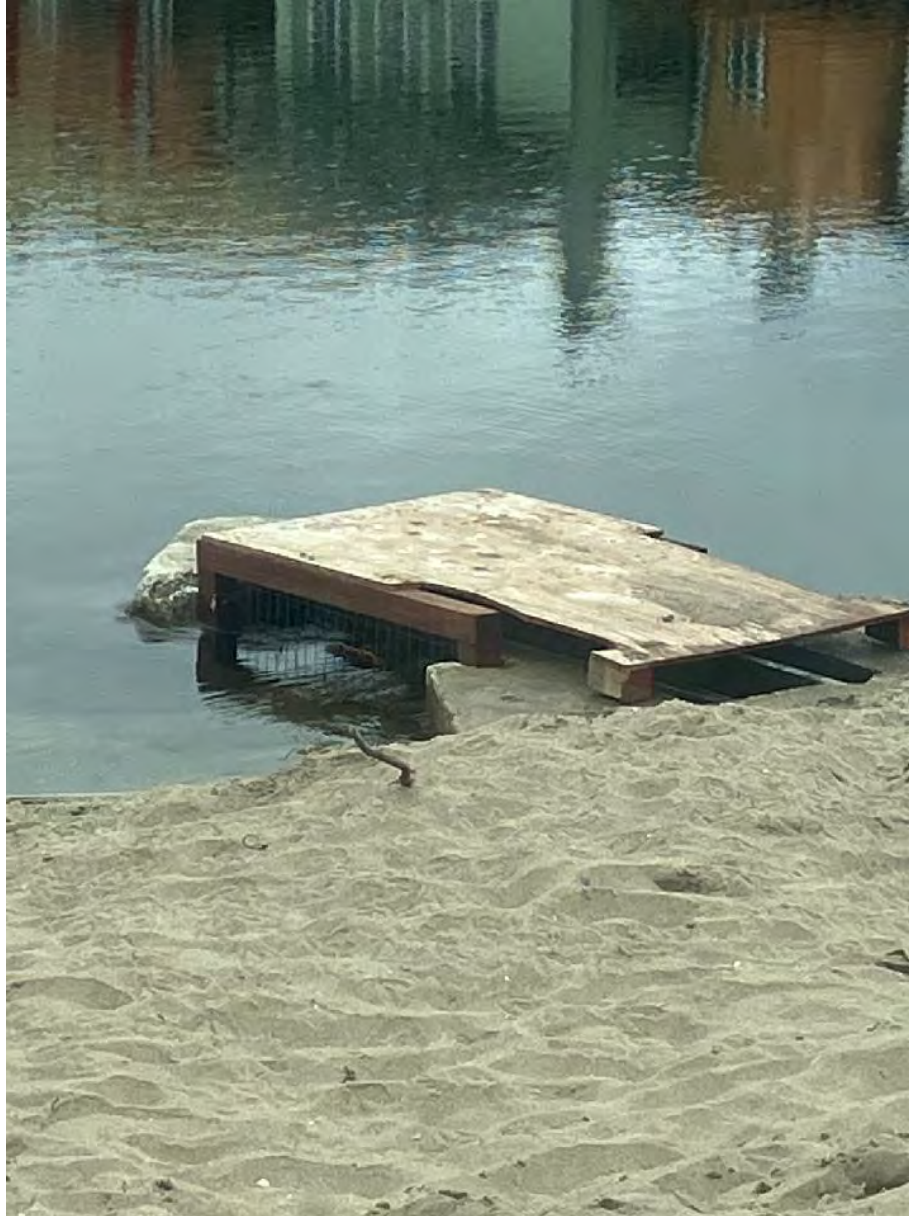
Flume inlet screen cleaned of debris. 31 May 2023
