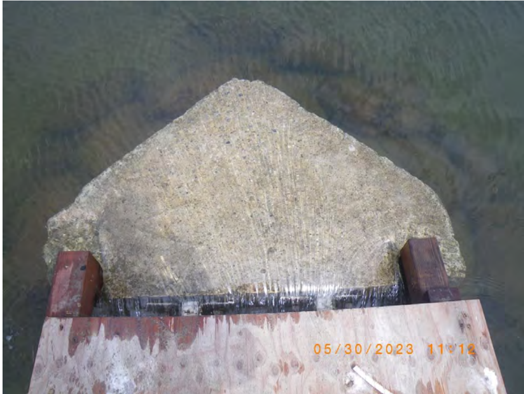
Steelhead smolt passage under the plywood cover at head of the flume. 30 May 2023. (The replacement stainless-steel grate was installed by 24 June 2023.)
