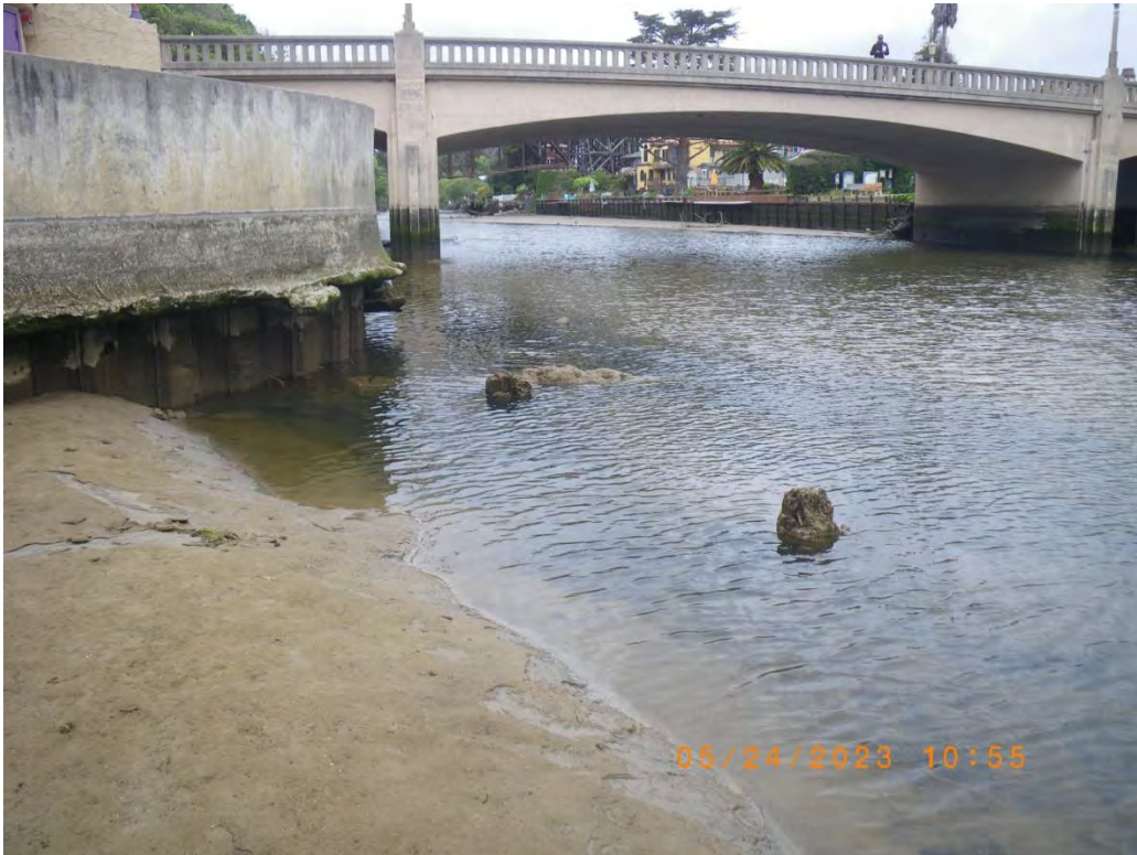
Deep hole beside Venetian Court wall. 24 May 2023
