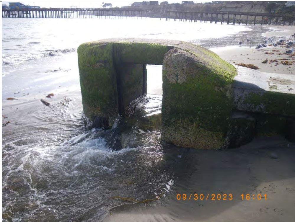
Flume outlet to the Capitola Beach and Monterey Bay. 30 September 2023
