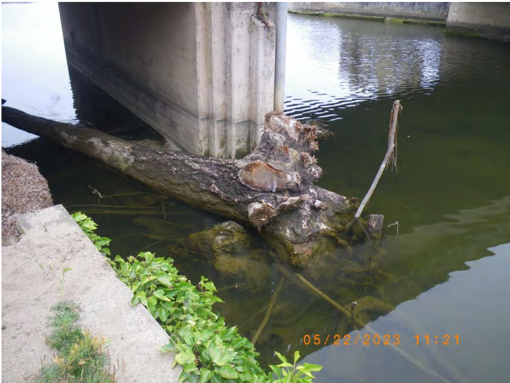
Log collected on Stockton Bridge abutment, offering fish cover. 22 May 2023
