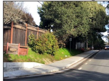
A newly completed sidewalk on Park Avenue
