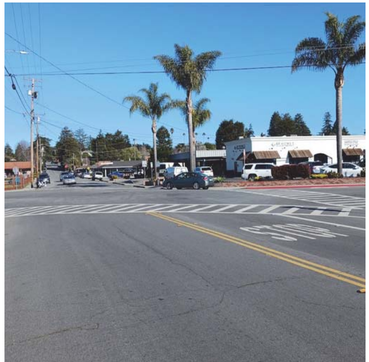
Image 4: Four way stop lacking bike facilities and modern pedestrian crossings at the intersection of Bay Ave and Capitola Ave. This area is known for higher ped/bike crashes.
