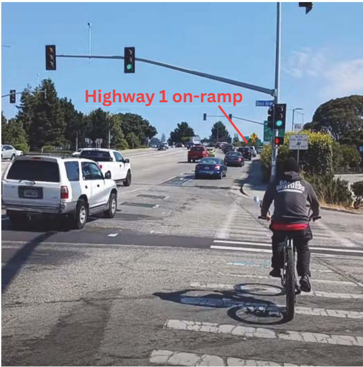
Image 1: Biker using crosswalk at the intersection at 41st Ave and Gross Rd. The bike lane is faded and unprotected and crosses into oncoming traffic at a Highway 1 on-ramp.
