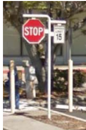
Typical sign design for on-site stop signs, speed limit signs, and other traffic control signage
