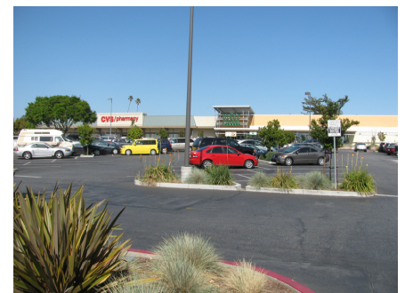
Variation in building setbacks (top and bottom) contribute to a lack of design coherence within the Plan area. Large parking lots fronting the street (bottom) contribute to the impression that the corridor is dominated by the automobile.
