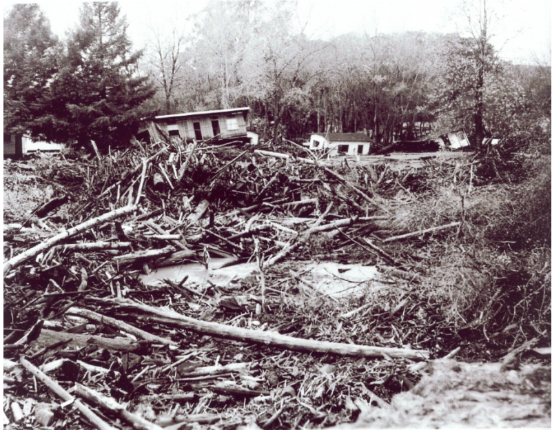
Figure 15 - Debris generated during the Flash Floods (ca. 1955)
