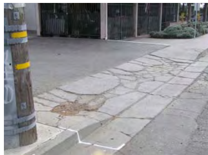
Large cracks in driveway
