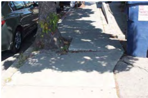
Sidewalk uplift due to tree roots.
