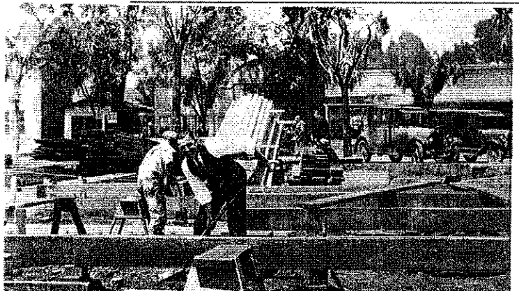
Orchestra leader Val Valente rolled his sleeves to help shovel dirt as construction began on the Big Top Ballroom. (Courtesy of the Macdonald family)
