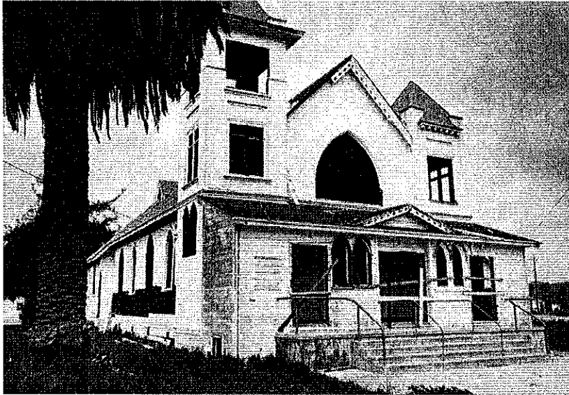
St. Joseph's Catholic Church, located at Bay and Capitola Avenues, was demolished in March 1973. ( Capitola Museum )
