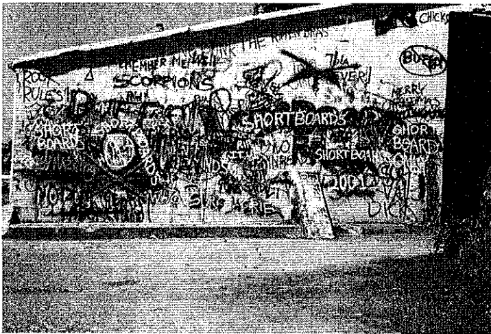
Capitola's sewer outfall was a 1933 WPA project. This photograph was taken shortly before the outfall was removed in the late 1980s. ( Capitola Museum )
