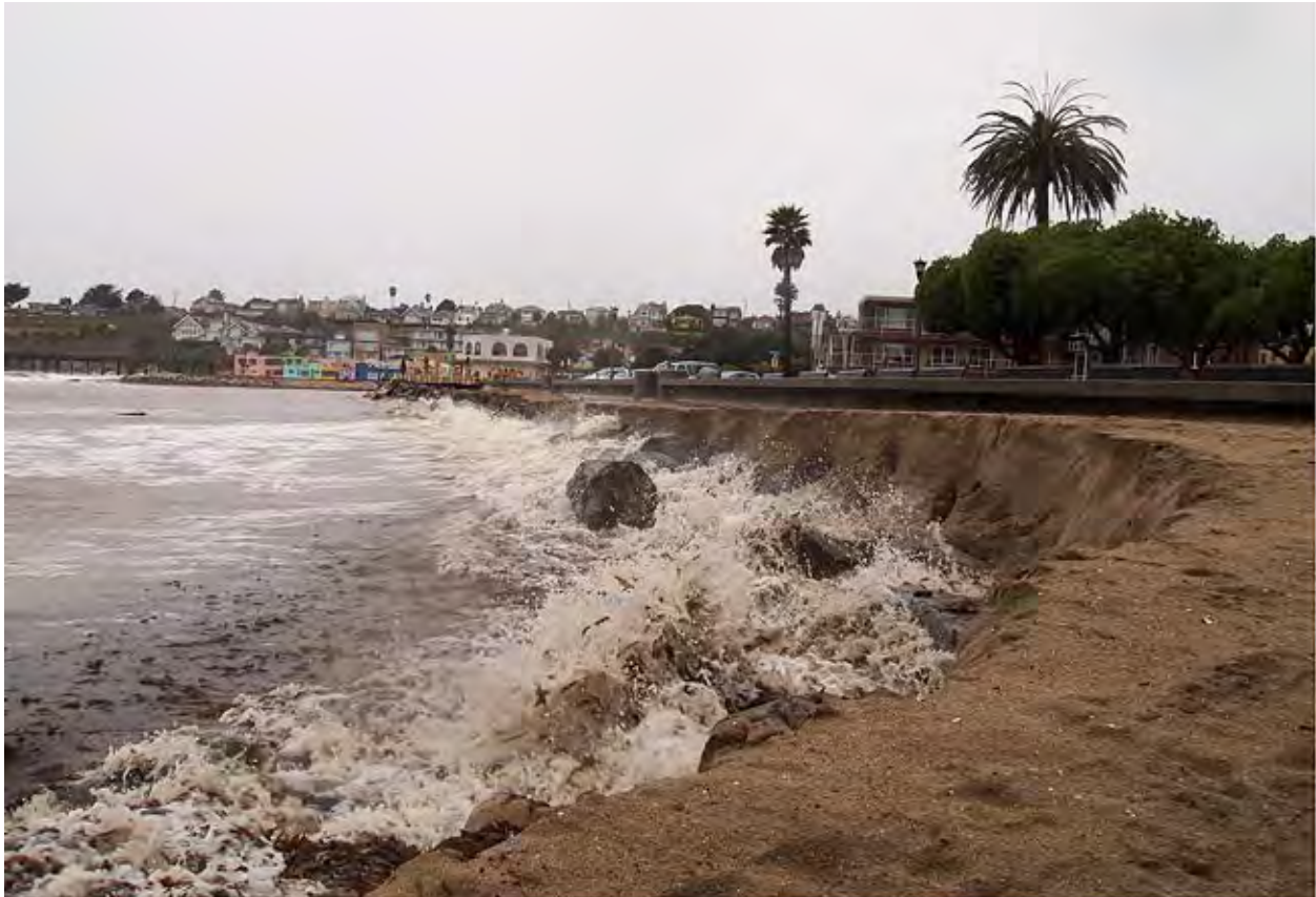
Figure 13 - Capitola Beach Erosion
