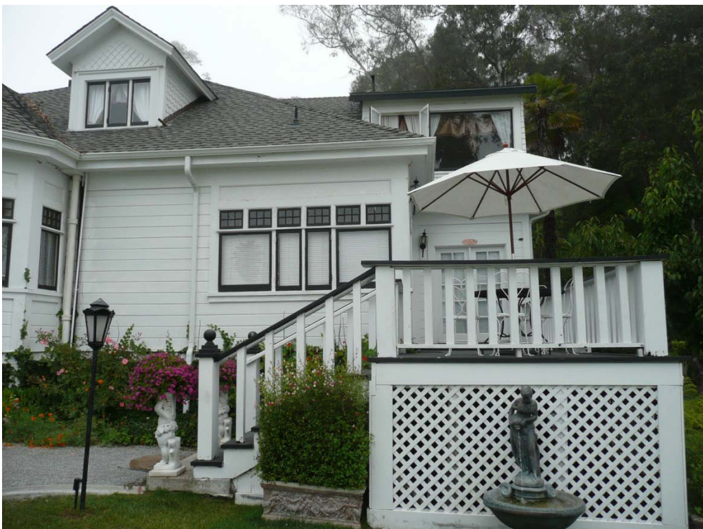
Main house, south elevation east porch, view looking north (Architectural Resources Group, July 2013)
