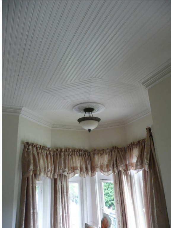
Main house interior, northeast corner bay window, view looking northeast (Architectural Resources Group, July 2013)
