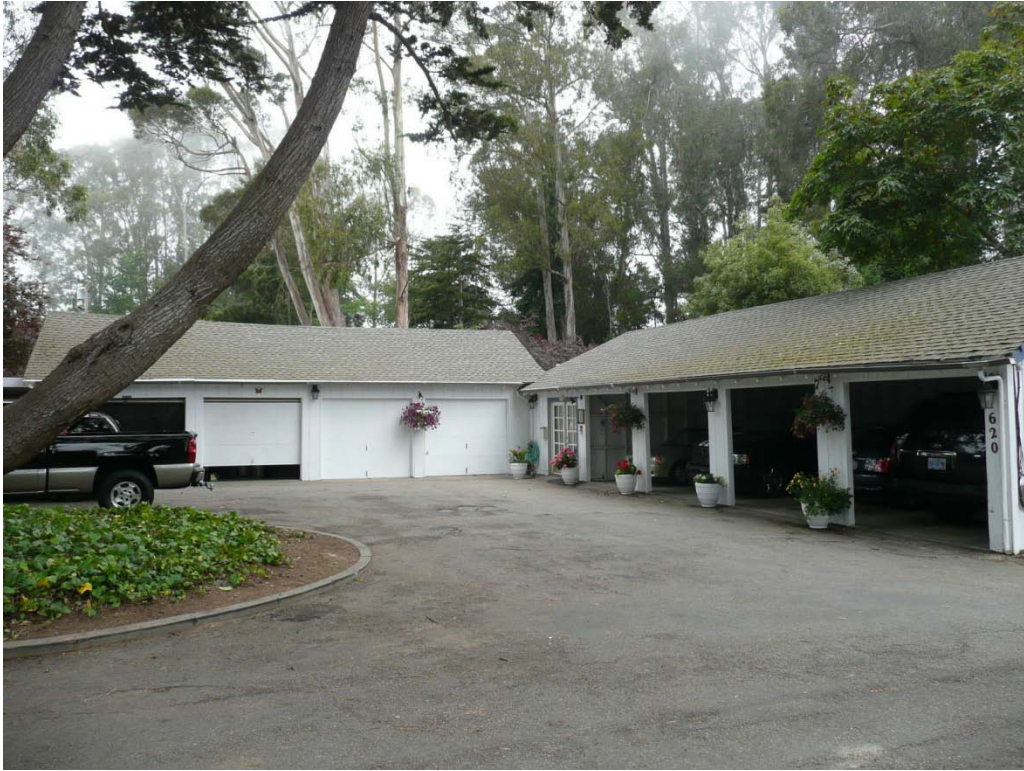
Garage/L-Shaped building, view looking north (Architectural Resources Group, July 2013)
