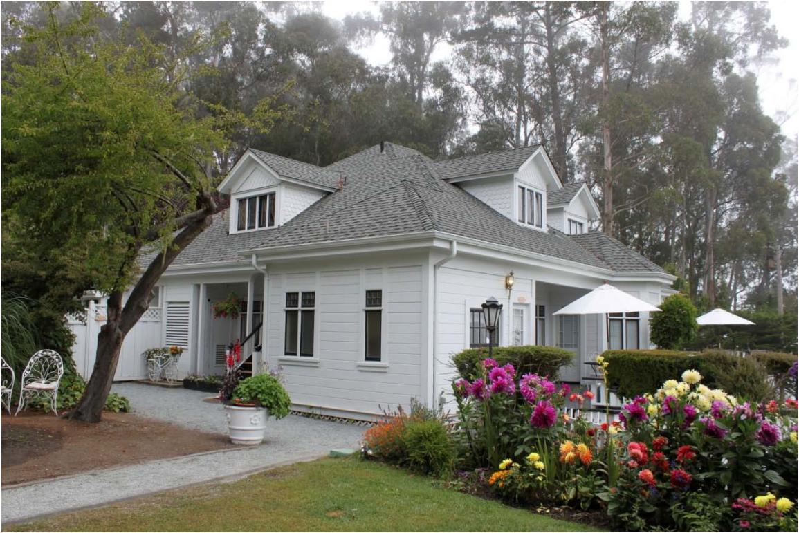
Main house, west and south elevations, view looking northeast (Architectural Resources Group, July 2013)
