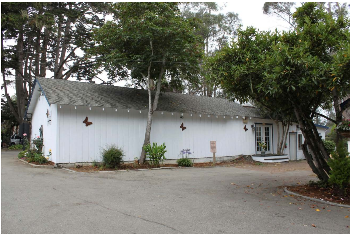
Garage/L-shaped building, east elevation, view looking west (Architectural Resources Group, July 2013)
