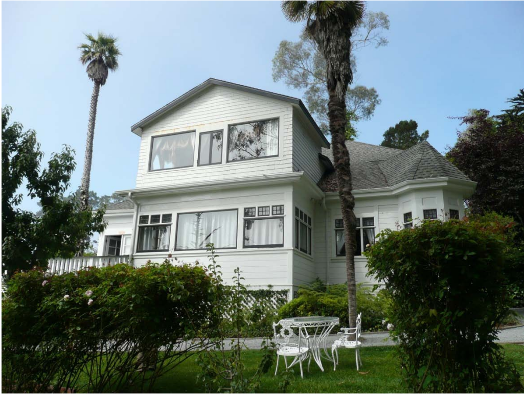
Main house, east elevation, view looking west (Architectural Resources Group, July 2013)
