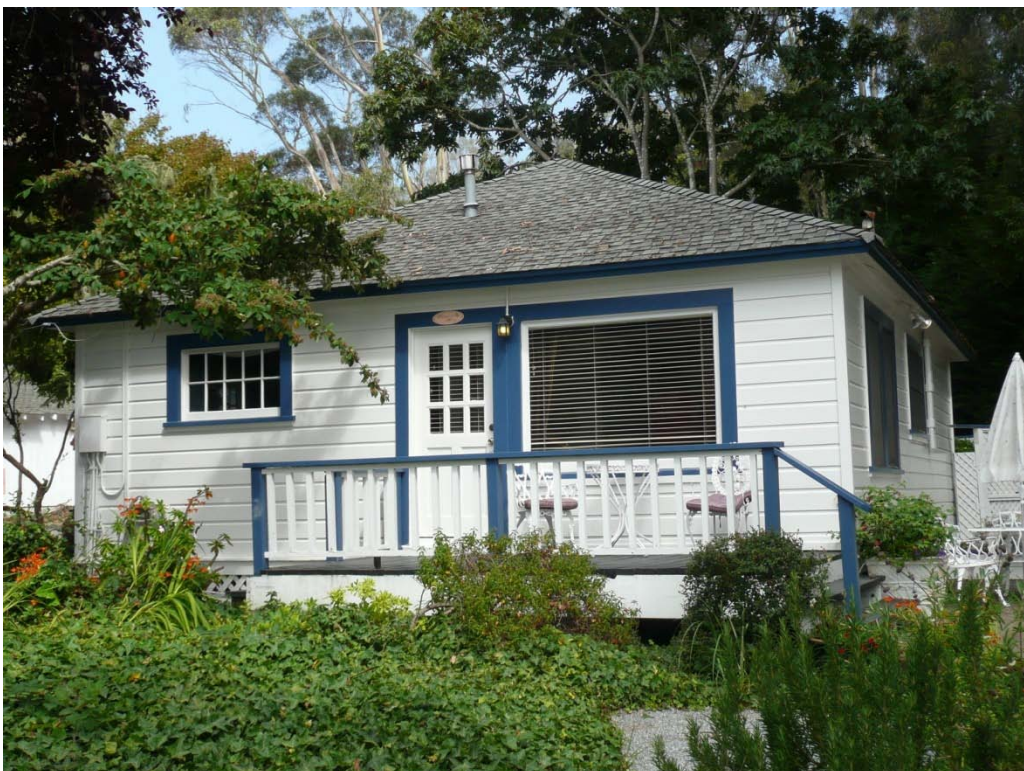
Cottage 1, south elevation, view looking north (Architectural Resources Group, July 2013)
