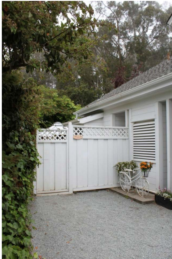
Main house, north end of west facade, view looking north (Architectural Resources Group, July 2013)
