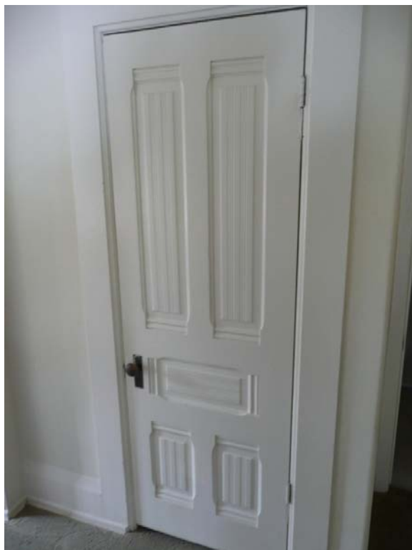
Example of doors located throughout Main house (Architectural Resources Group, July 2013)
