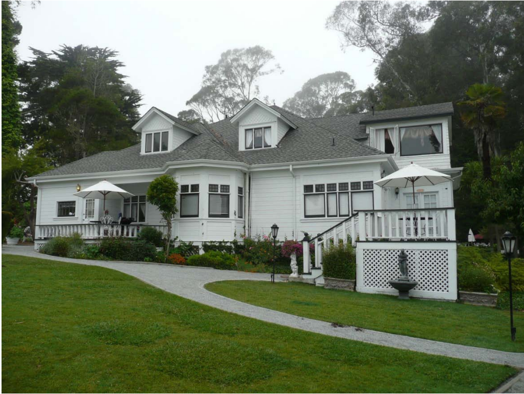
Main house, south elevation, view looking north (Architectural Resources Group, July 2013)
