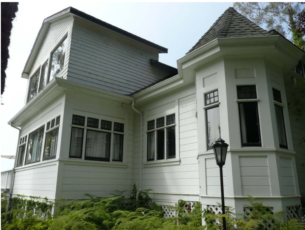
Main house, east elevation, view looking southwest (Architectural Resources Group, July 2013)
