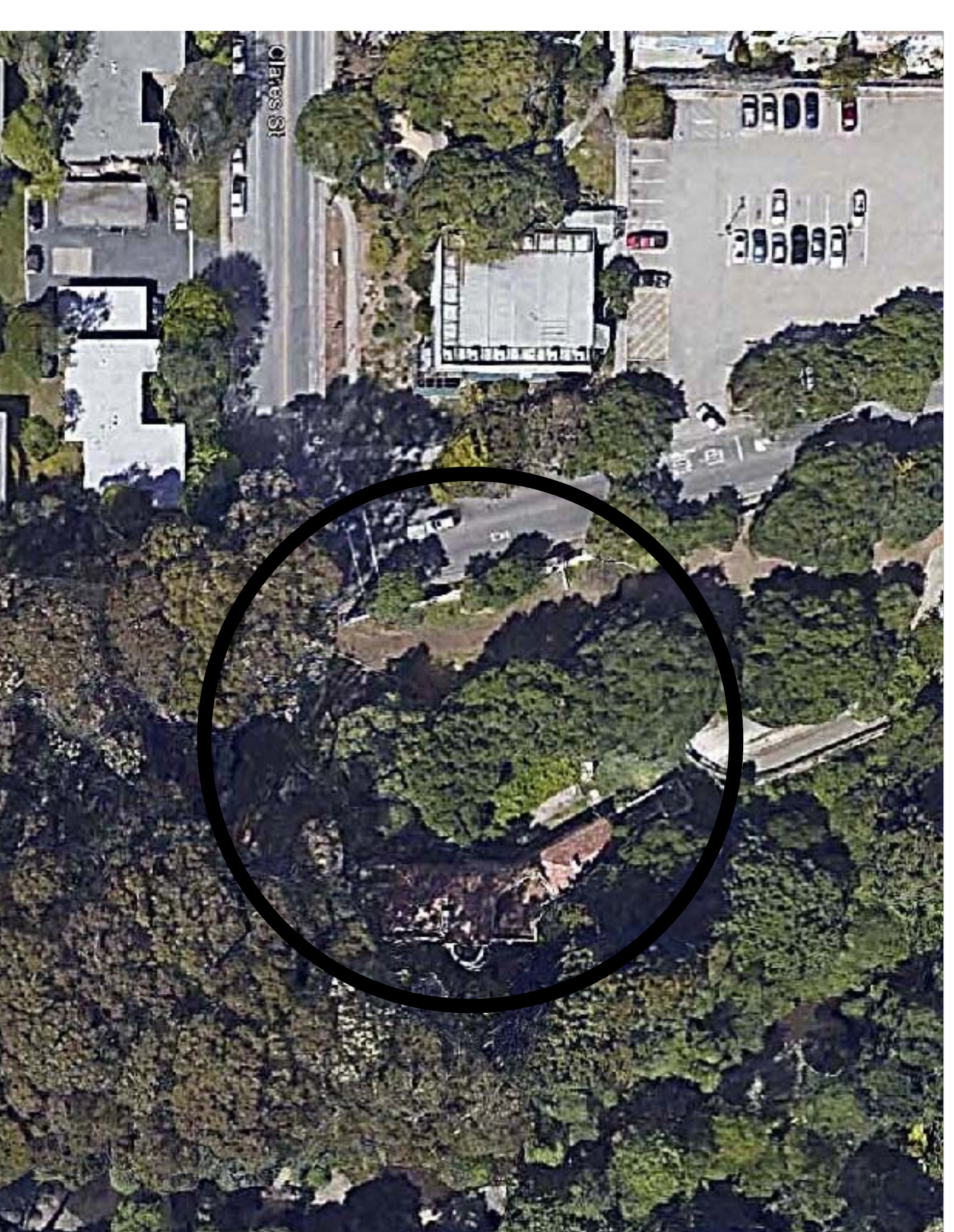
Clares Street and Wharf Road
