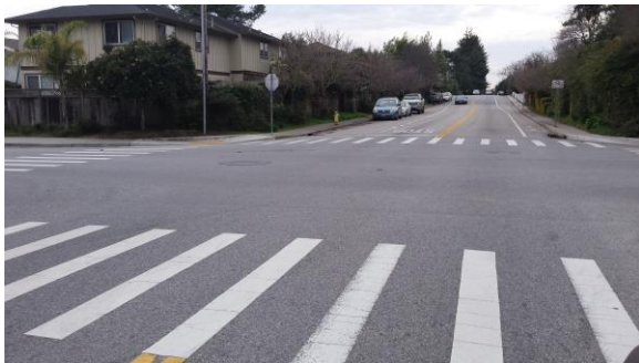
38 th Avenue intersection in good condition.
