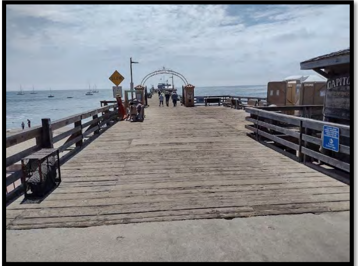
Photo Point 2 – Base of Wharf
