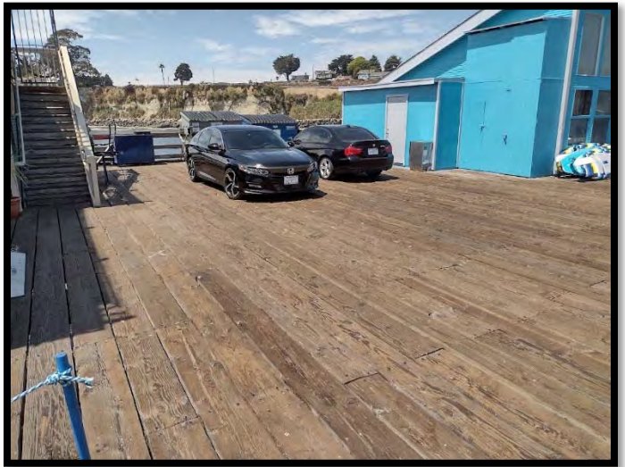
Photo Point – 4 Deck Repair Area
