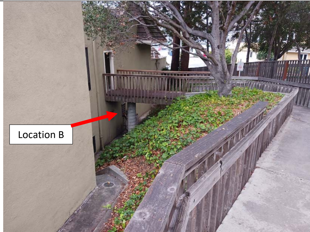
Location B – Electrical Room
