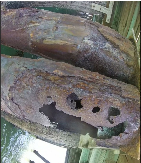
PHOTO 6 STEEL PILES - BENT 75F
