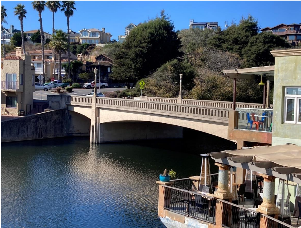
Figure 1. Stockton Avenue Bridge, view towards West.
