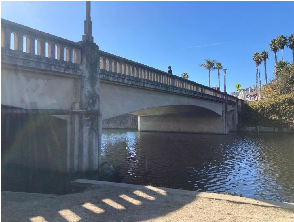
Figure 2. Stockton Avenue Bridge, view towards Southwest.
