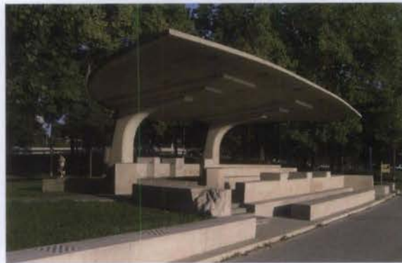
Figure 8. The Chess Pavilion in Chicago's Lincoln Park was designed by architect Morris Webster and constructed in 1956. The pavilion is a distinctive landscape feature, with its reinforced concrete cantilevered slab that provides cover for chess players.
