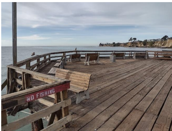
View from the front of Capitola Wharf
