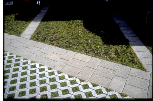
Examples of Permeable Pavement Interlocking/Porous pavers and turf block
