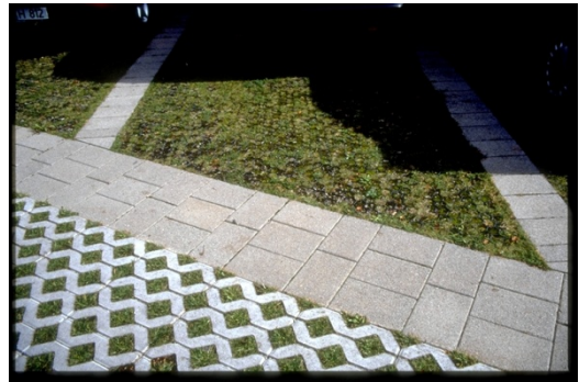
Figure 2: Examples of Permeable Pavement
