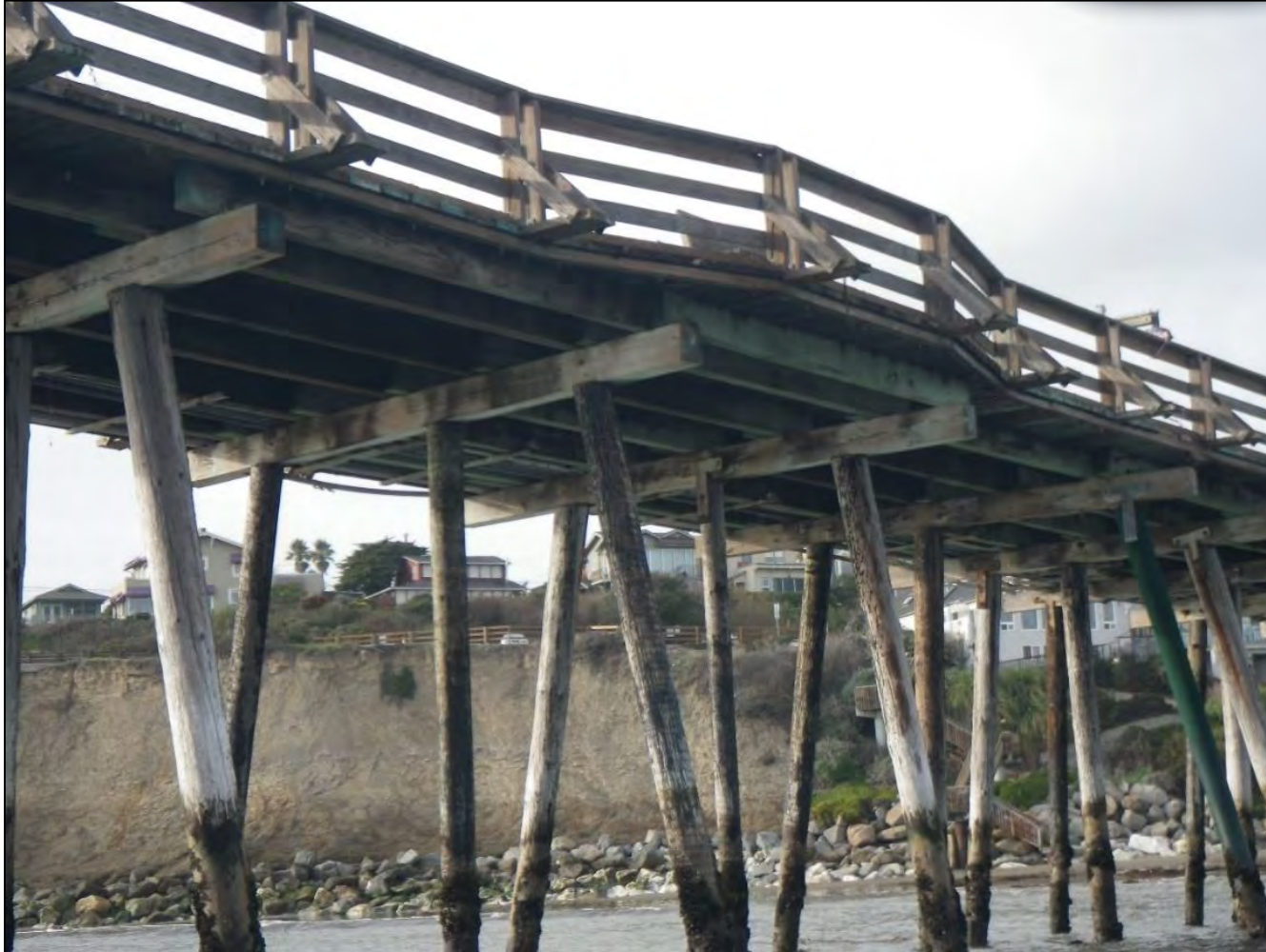
Photo 2. Typical Wharf Structural Framing.
