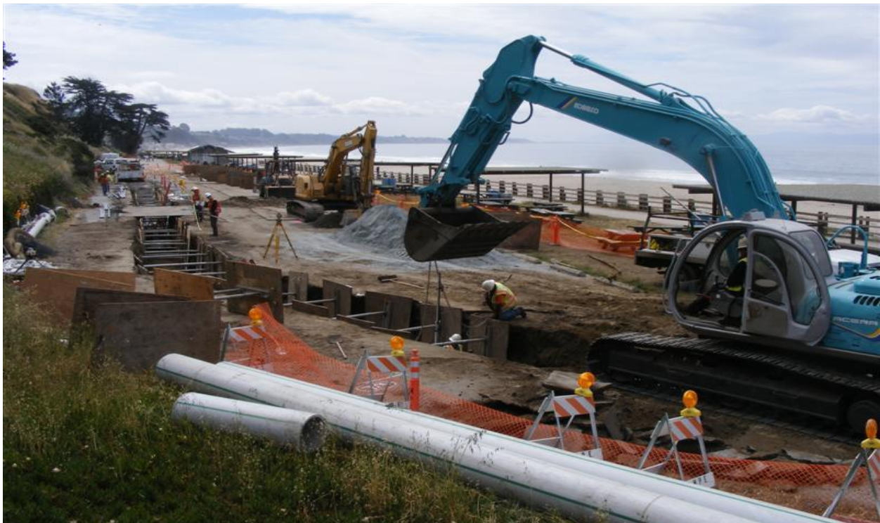
Aptos Sewer Transmission Main Relocation – Seacliff State Beach (2010)
